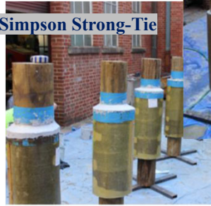
Repaired timber piles
