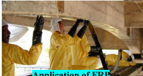
Application of FRP
