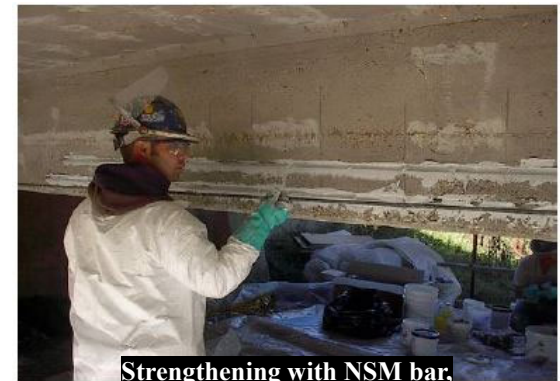
Strengthening with NSM bar, (Aiswarya and Prabhakaran, 2017)
