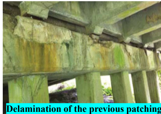
FRP-repair of the Morganza Spillway bridge pile cap, Louisiana [Gopu and Balaguru 2016]
