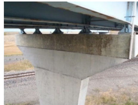
Bridge #01490, bent cap repair
