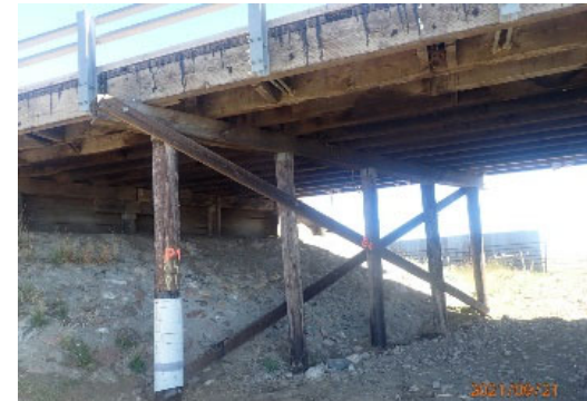
Bridge #06131, Bottom 4ft of Bent 4 Pile 1 was FRP repaired.
