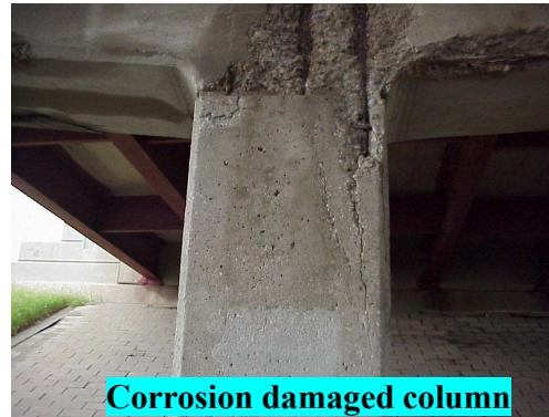
Repair of corrosion-damaged columns, Michigan [Harichandran and Baiyasi 2000]
