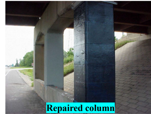
Repair of corrosion-damaged columns, Michigan [Harichandran and Baiyasi 2000]
