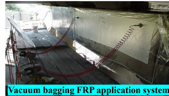
FRP jackets for deteriorating pier cap of Silver Spring Cove Bridge, Rhode Island [Balaguru and Lee 2005]
