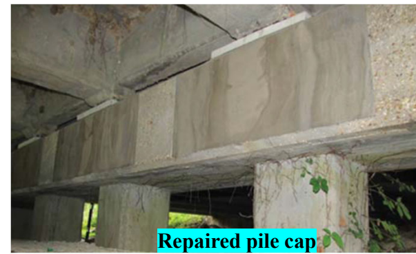
FRP-repair of the Morganza Spillway bridge pile cap, Louisiana [Gopu and Balaguru 2016]
