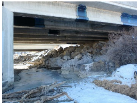
Bridge #01044, girder repair
