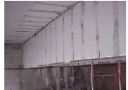
Repair of Route 378 Bridge, New York
