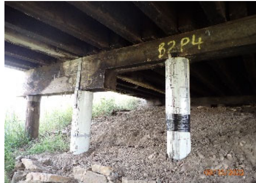
Bridge #02568, Piles 4 and 5 of Bent 2 were FRP wrapped for full height.
