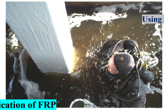
Corrosion repair of submerged concrete piles of Friendship trail bridge, Florida [Sen and Mullins 2007]
