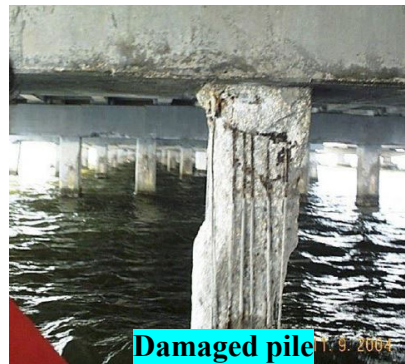
Corrosion repair of submerged concrete piles of Friendship trail bridge, Florida [Sen and Mullins 2007]
