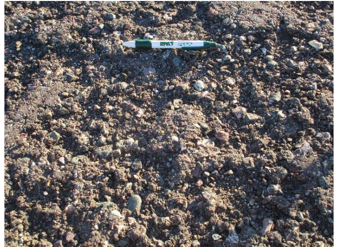
A-1, Surface detail with high raveling
