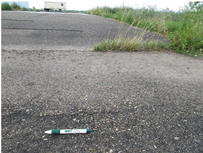
T-4, Surface detail with depression
