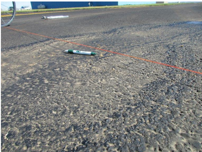
T-2, Surface detail with depression
