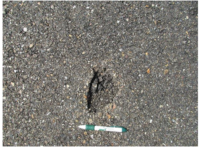
R-1, Surface detail with gouge
