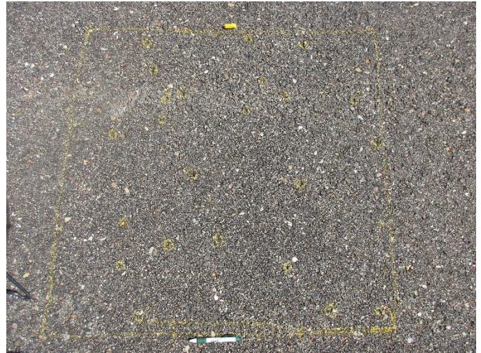
A-1 , Surface detail with medium raveling count
