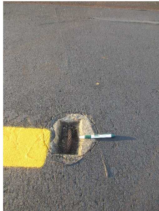
A-1B, Surface detail with tie down
