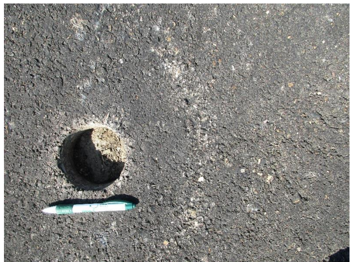
R-1 , Surface detail with open core hole
