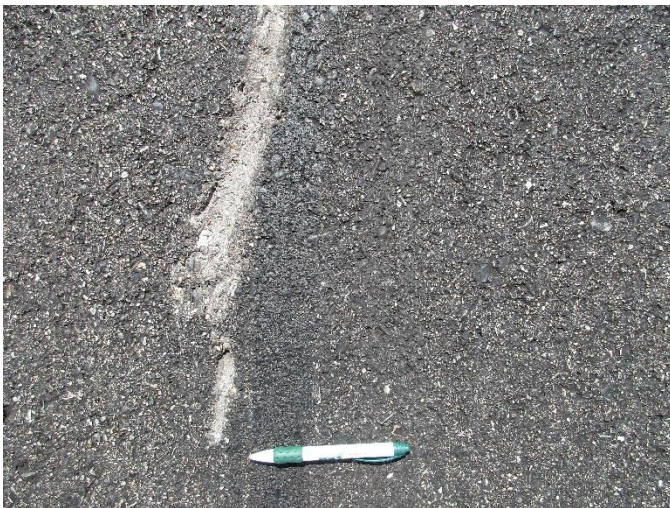
R-3, Surface detail with gouge
