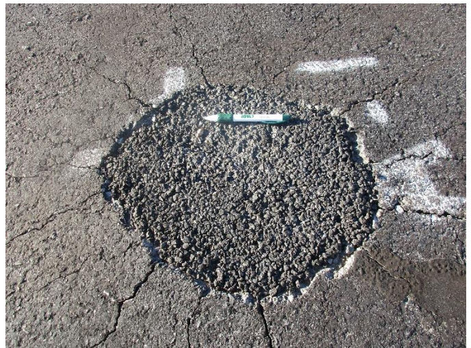
T-2 , Surface detail with swelling & bore hole
