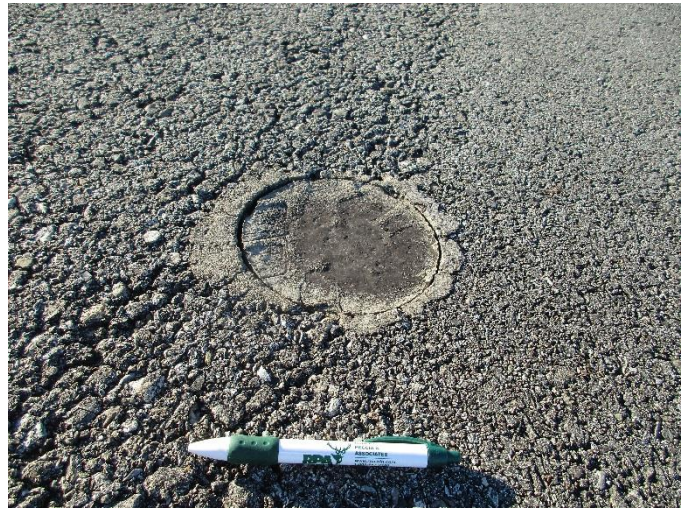
R-11, Surface detail with bore hole
