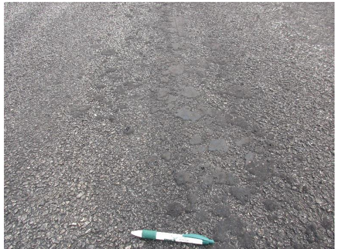
T-5, Surface detail with bleeding
