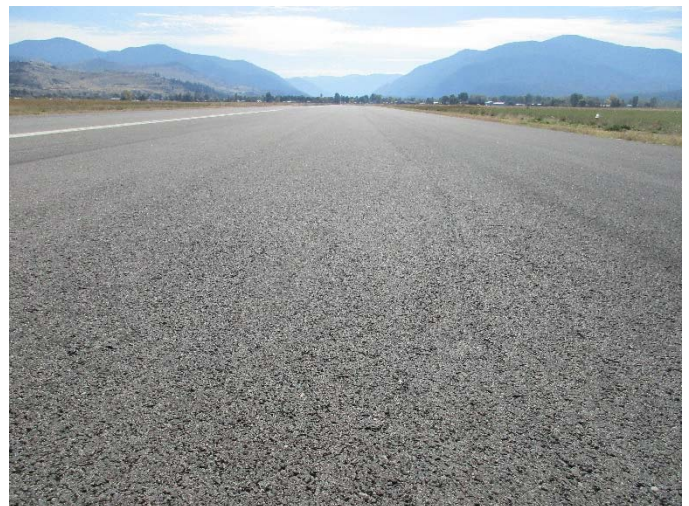
R-1 , Pavement overview
