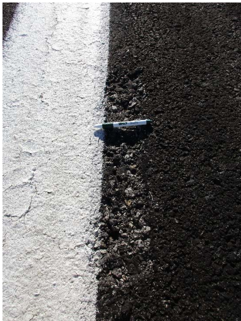
R-2, Surface detail with raveling
