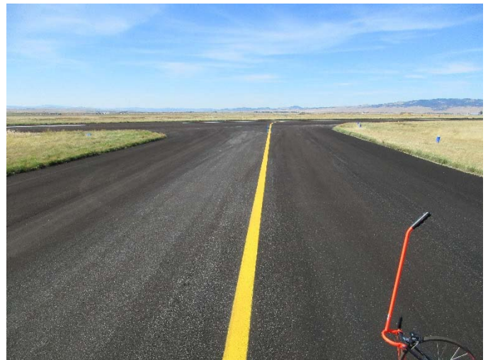
T-12 , Overview with fresh seal coat
