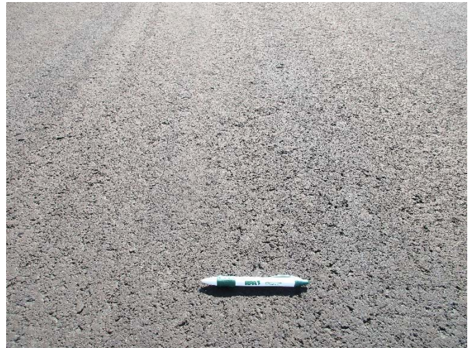
R-12 , Surface detail with seal coat
