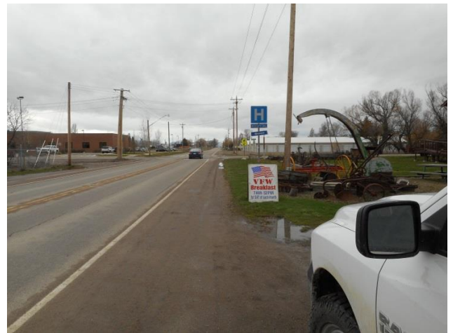
Section 2- Looking west in front of Museum of the Rockies
