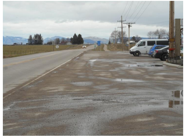
Section 2 – Looking west in front of Westland Seed at the existing multi-use path
