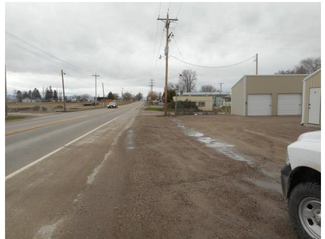
Section 2 – Looking west directly across from St. Luke Hospital
