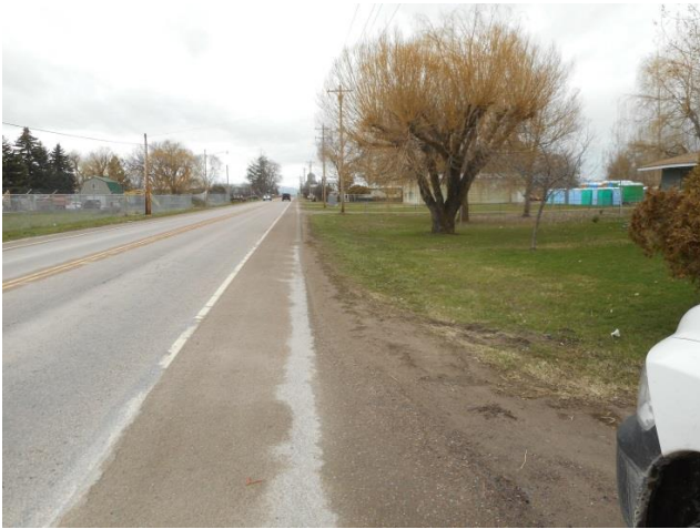
Section 2 – Looking west towards Acre Lawn Ct.
