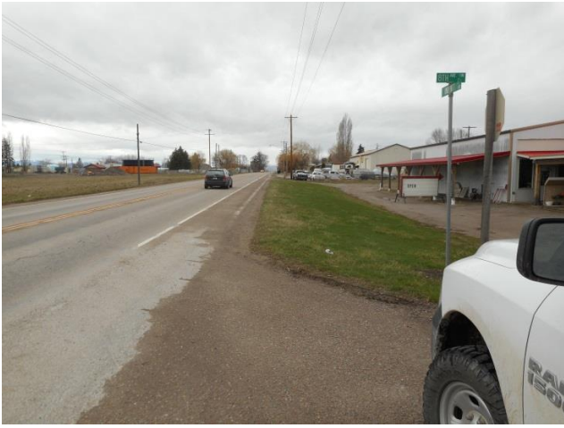
Section 2 – Looking west at 8 th Avenue NW
