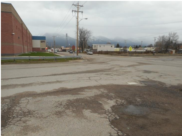
Start of Section 2 – Looking east across 3 rd Avenue NW
