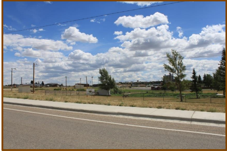
Existing Sidewalk on Skyland Road
