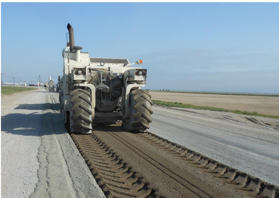
Exhibit 6-4 Pavement Pulverization
