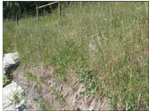
Photo 5 Description: Coir and bank vegetation establishment. Compass: 330 (North-Northwest)
