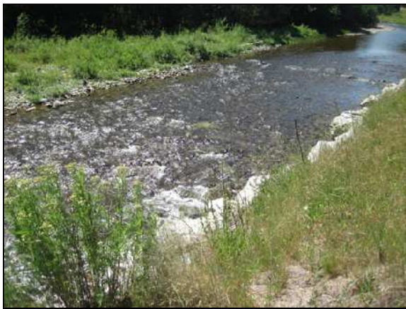
Photo 7 Description: Upstream view of both j-hook vanes. Compass: 230 (Southwest)
