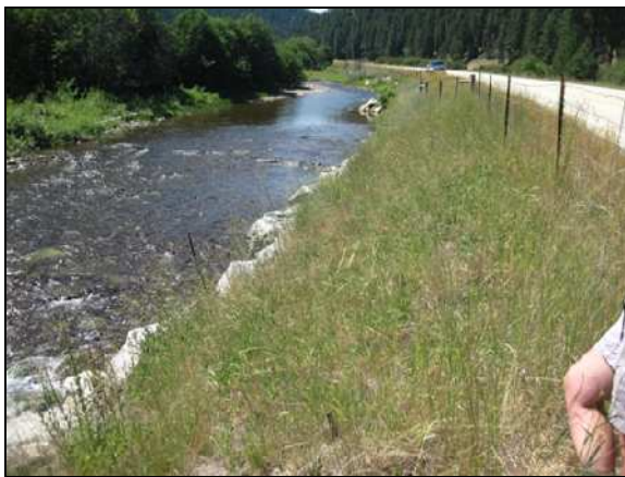
Photo 8 Description: Upstream j-hook vane. Compass: 270 (West)
