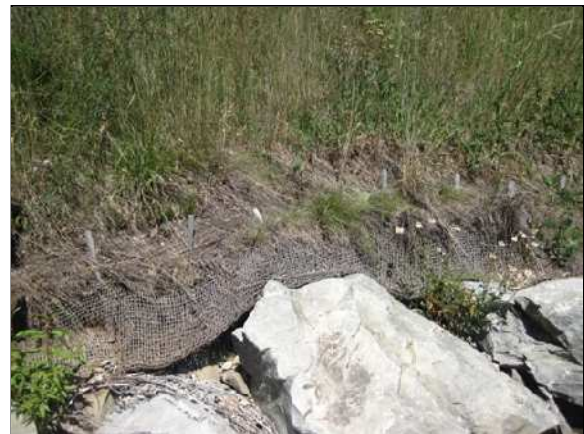
Photo 6 Description: Coir fabric above riprap. Compass: 0 (North)
