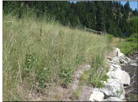
Photo 4 Description: Downstream extent of riprap and coir. Compass: 40 (Northeast)
