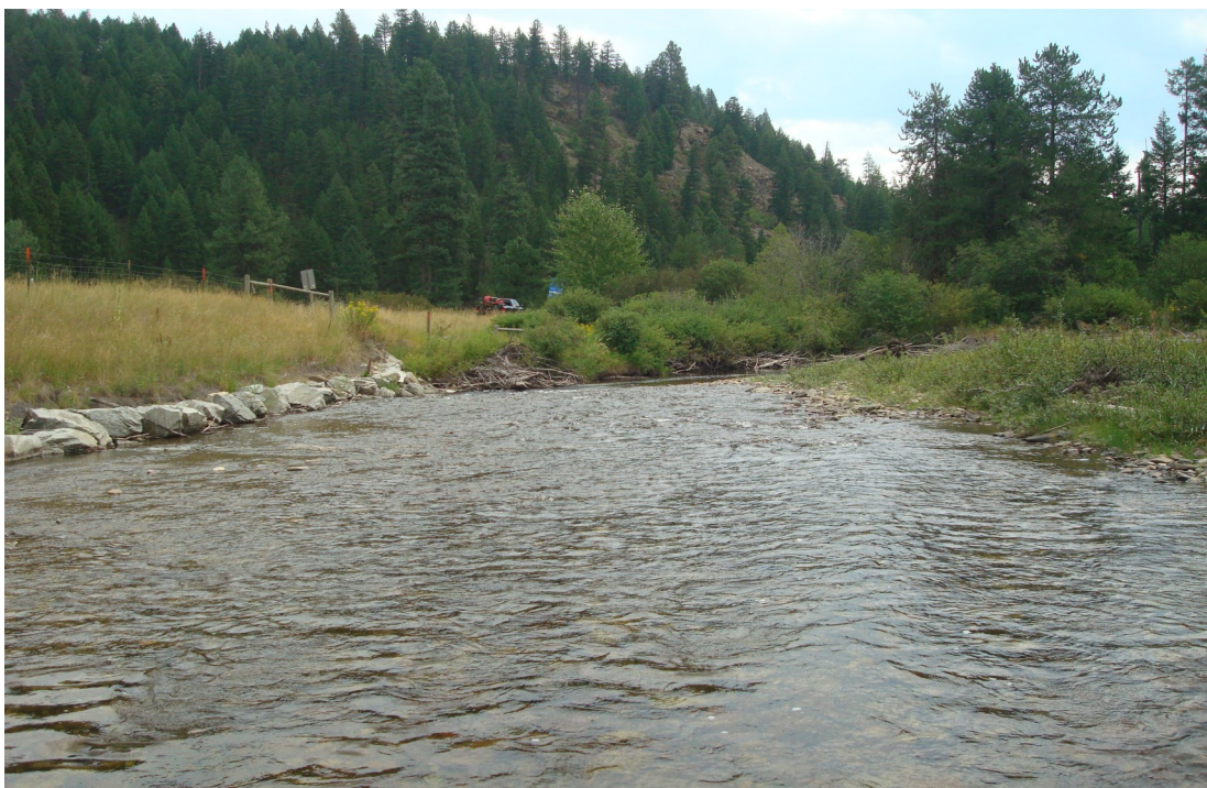
In Channel Looking Downstream A-6
