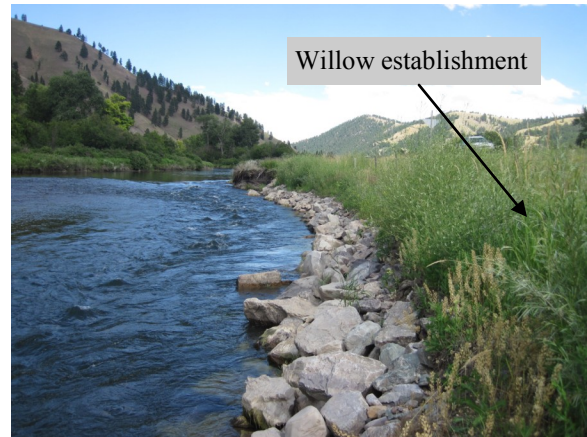
Photo 1 Description: View upstream looking at revetment. Taken in 2014
