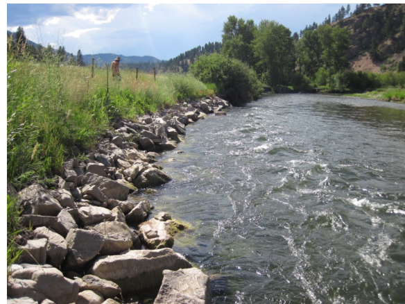
Photo 9 Description: Looking downstream at revetment. Taken in 2014
