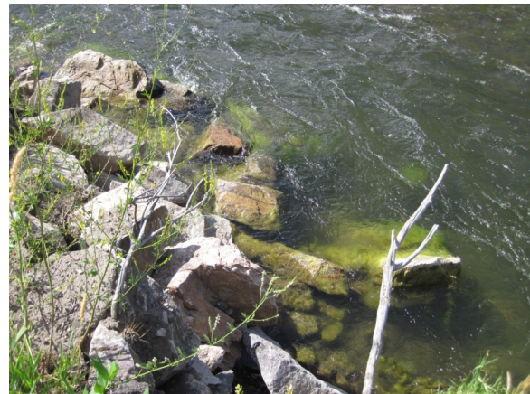
Photo 11 Description: Upstream extent of rip-rapped stream-bank. Taken in 2014
