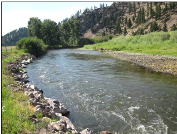
Photo 13 Description: Looking downstream at revetment Taken in 2013
