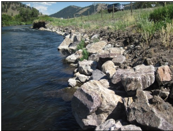
Photo 2 Description: Toe of revetment looking upstream. Taken in 2013
