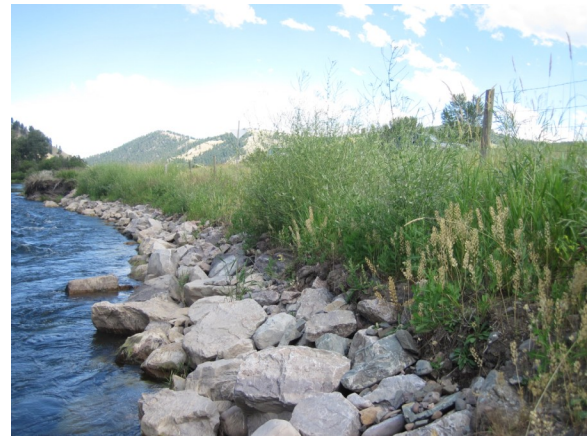
Photo 2 Description: Toe of revetment looking upstream. Taken in 2014
