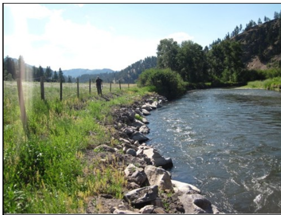
Photo 9 Description: Looking downstream at revetment. Taken in 2013
