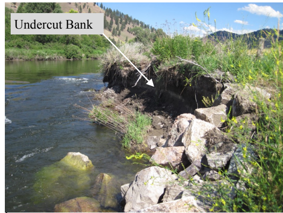
Photo 7 Description: Eroding streambank at upstream extent. Taken in 2014
