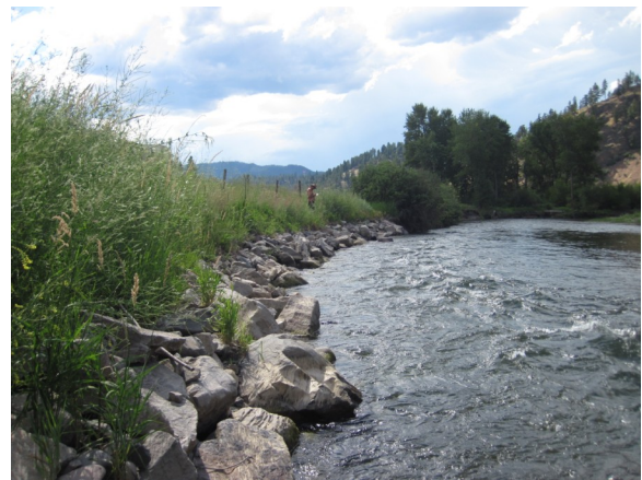
Photo 13 Description: Looking downstream at revetment. Taken in 2014
