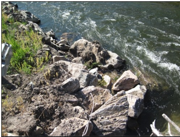
Photo 11 Description: Upstream extent of rip-rapped stream-bank. Taken in 2013
