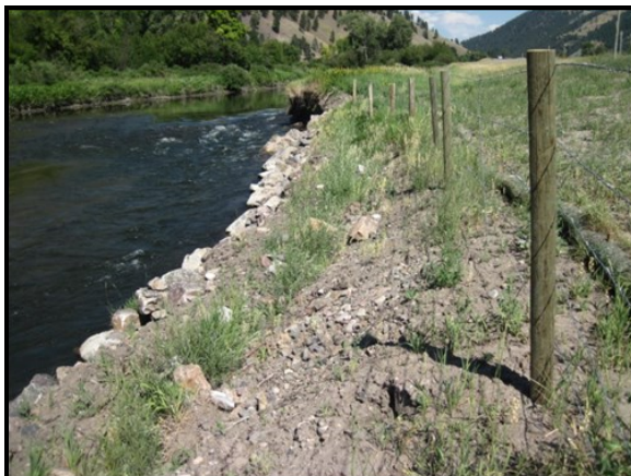
Photo 3 Description: Middle of revetment looking upstream. Taken in 2013
