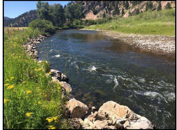
Photo 13 Description: Looking downstream at revetment. Taken in 2016
