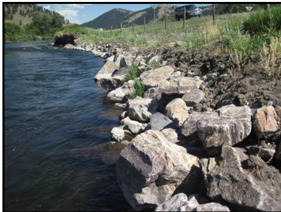
Photo 2 Description: Toe of revetment looking upstream. Taken in 2013
