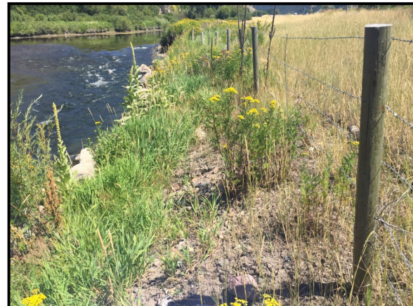
Photo 3 Description: Middle of revetment looking upstream. Taken in 2016
