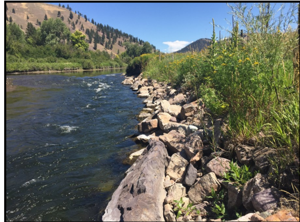
Photo 2 Description: Toe of revetment looking upstream. Taken in 2016
