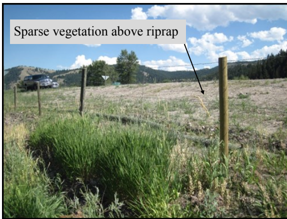
Photo 5 Description: Highway embankment / access area. Taken in 2013
