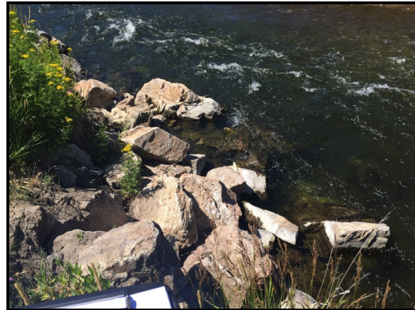
Photo 11 Description: Upstream extent of rip-rapped stream-bank. Taken in 2016
