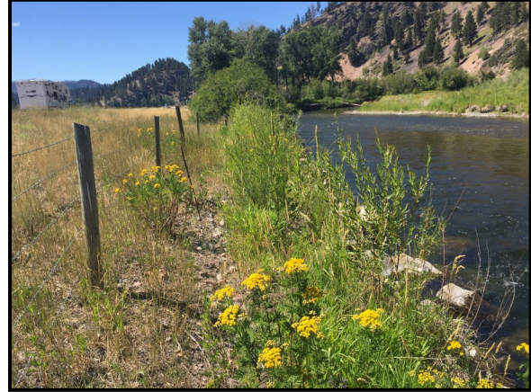
Photo 8 Description: Middle of revetment looking downstream. Taken in 2016
