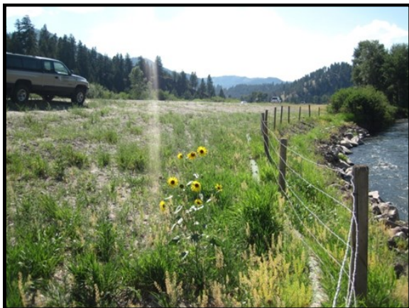
Photo 12 Description: Highway embankment adjacent to bank. Taken in 2013
