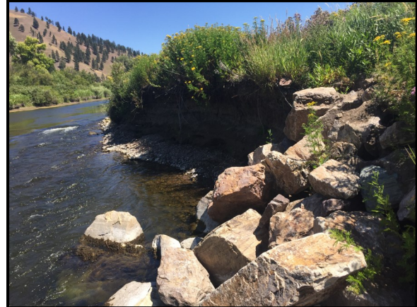
Photo 7 Description: Eroding streambank at upstream extent. Taken in 2016
