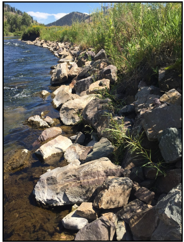
Additional Photo 2 Description: Willow growing in revetment Taken in 2016
