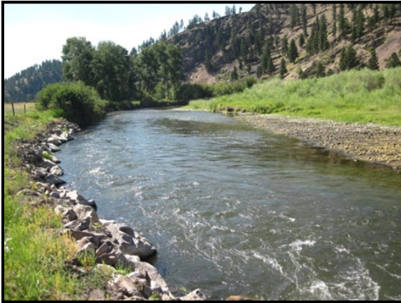
Photo 13 Description: Looking downstream at revetment Taken in 2013
