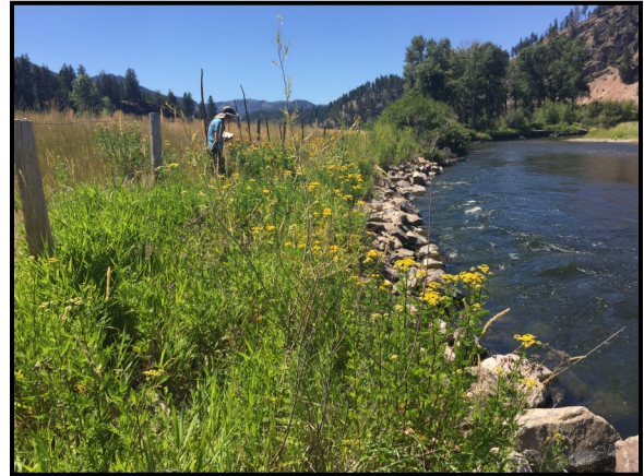
Photo 9 Description: Looking downstream at revetment. Taken in 2016
