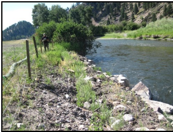
Photo 8 Description: Middle of revetment looking downstream. Taken in 2013
