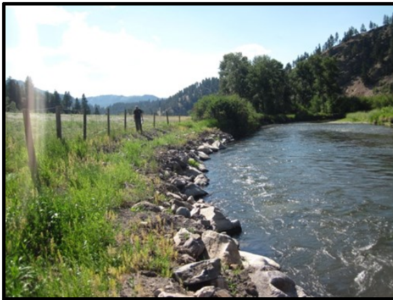
Photo 9 Description: Looking downstream at revetment. Taken in 2013
