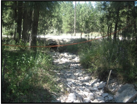
Photo Point 1.1—2013 Description: View of tributary/culvert entering from west. Compass: 270 (West)
