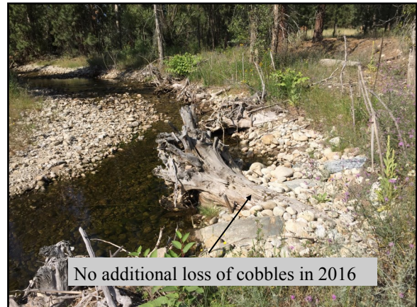
Additional Photo 1—2016 Description: Root wads upstream of bridge.
