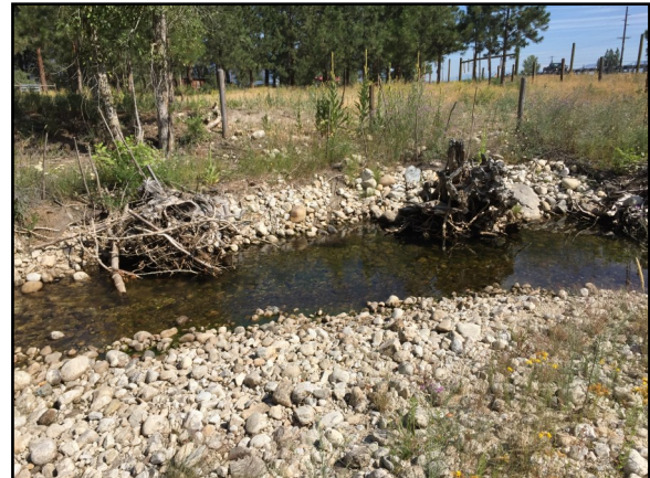
Additional Photo 2—2016 Description: Root wads upstream of bridge.
