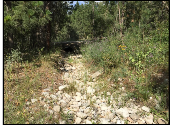
Photo Point 1.1—2016 Description: View of tributary/culvert entering from west. Compass: 270 (West)
