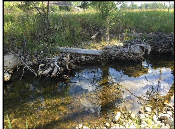
Photo Point 4.2—2016 Description: View of root wads on north bank downstream of bridge. Compass: 0 (North)
