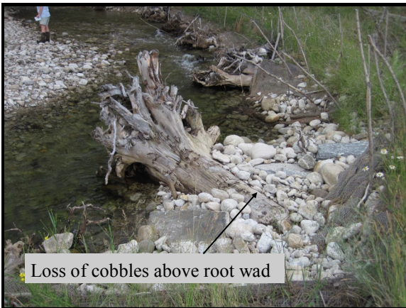
Additional Photo 1—2014 Description: Root wads upstream of bridge.
