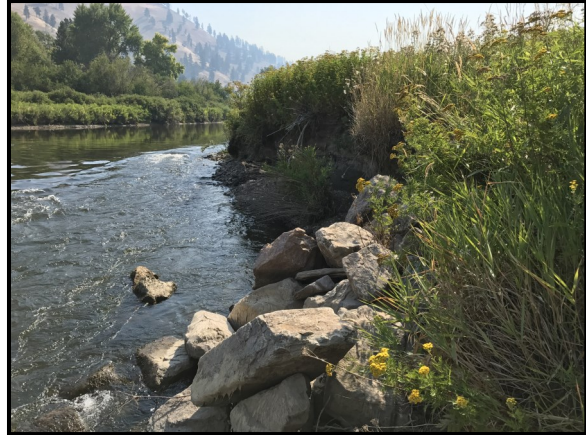
2013 2017 Photo 7: Eroding streambank at upstream extent of stabilized bank
