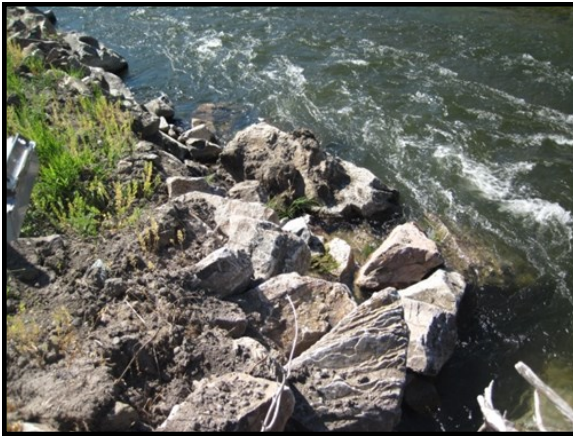
2013 2017 Photo 10: Upstream extent of riprapped stream bank.
