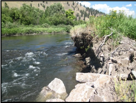
2013 2017 Photo 7: Eroding streambank at upstream extent of stabilized bank
