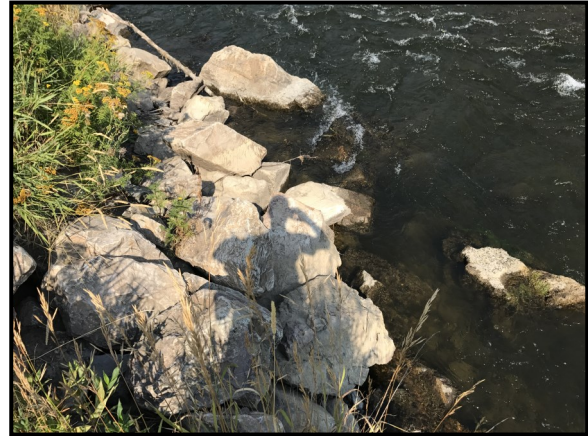
2013 2017 Photo 10: Upstream extent of riprapped stream bank.
