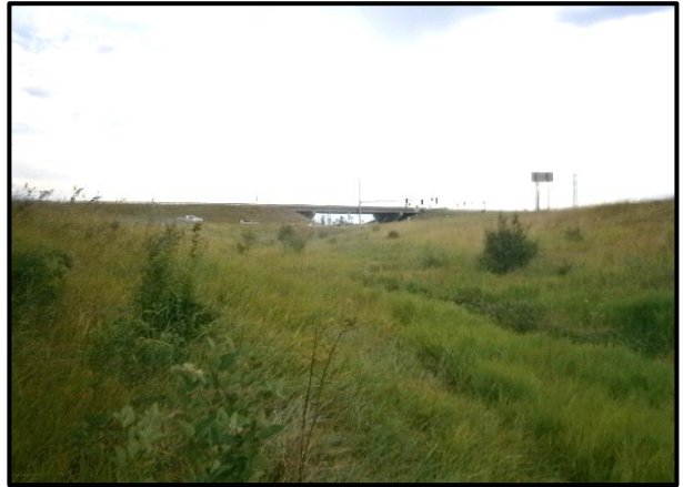
Survey Photo 28: T4 Left looking east downstream.
