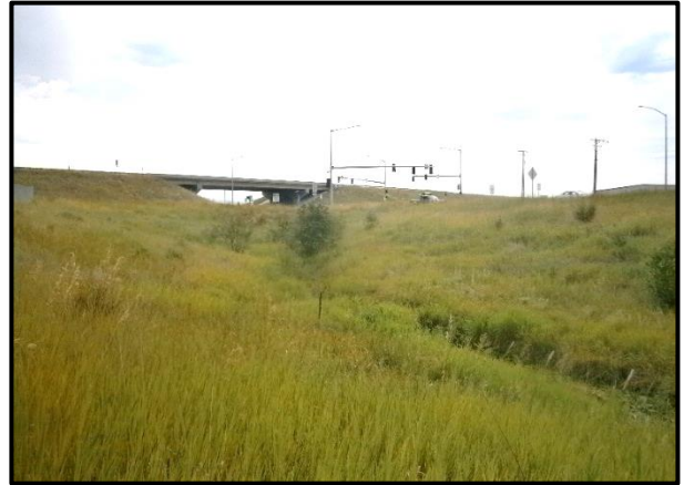
Survey Photo 20: T3 Left looking east downstream.
