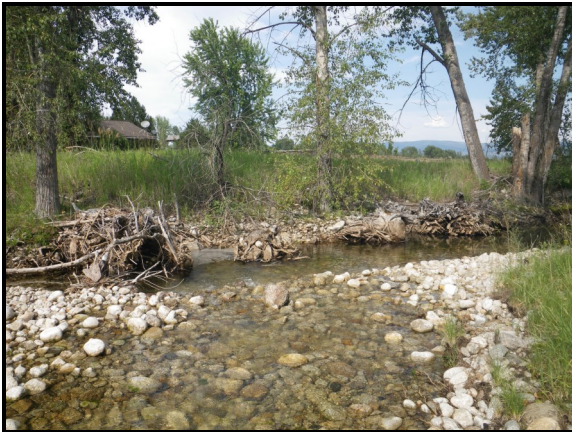
Additional Photo 1: Looking downstream at exposed root wads on the left bank at the downstream end of the project area.
