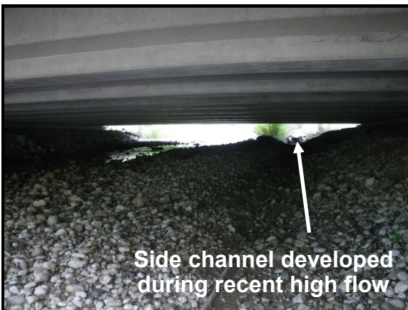
Additional Photo 5: Looking upstream under the bridge at recently deposited gravel and cobble and the side channel that developed during recent high flows.
