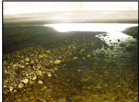
Additional Photo 4: Looking downstream at gravel and cobble recently deposited under the bridge.
