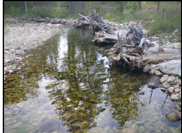
Additional Photo 2: Looking upstream at exposed root wads on the left bank upstream of the bridge where increased scour was observed in 2020
