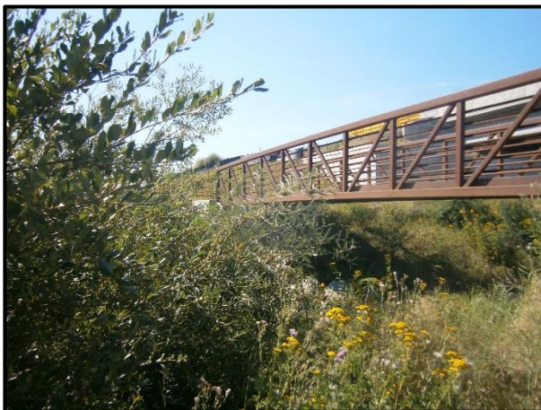
Survey Photo 23: T4 Left: Looking South to T4 Right.
