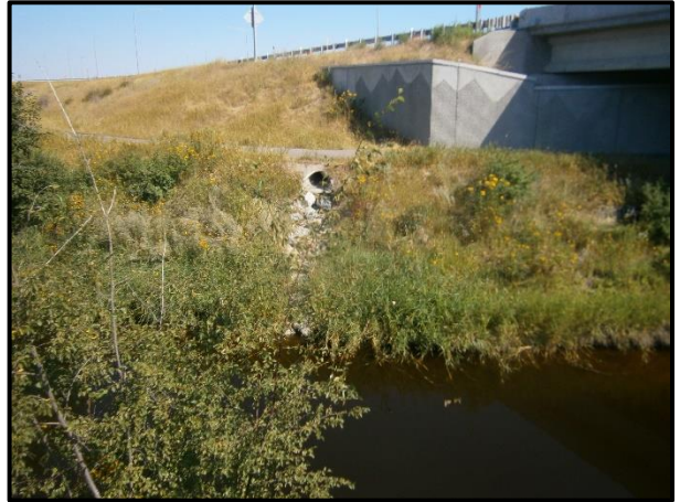
Survey Photo 8: T2 Right: Looking North to T2 Left.
