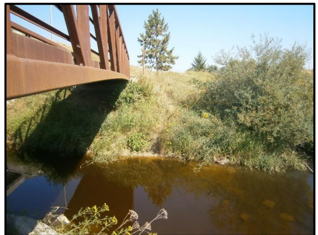
Survey Photo 24: T4 Right: Looking North to T4 Left.
