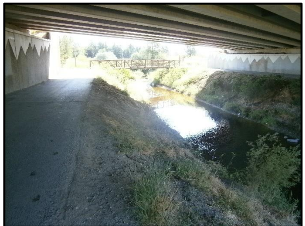
Survey Photo 18: T3 Left: Looking East downstream.
