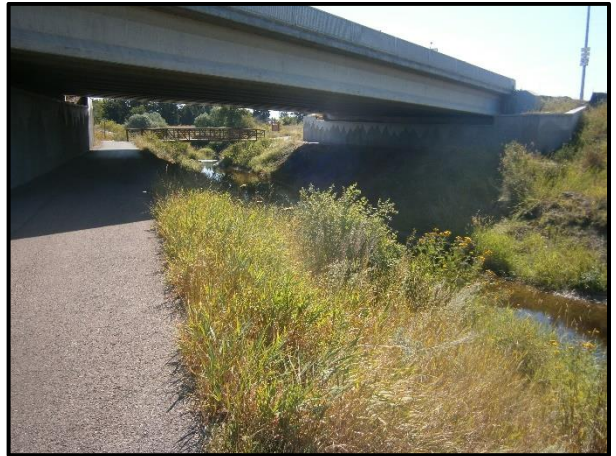
Survey Photo 10: T2 Left: Looking East downstream.
