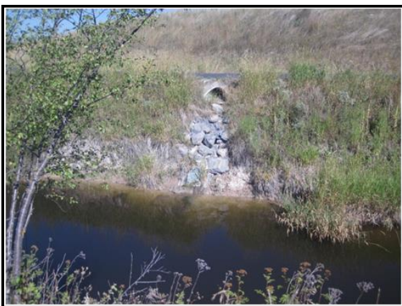
Additional Photo 6: Stabilized culvert outlet on the upstream end of the project area.
