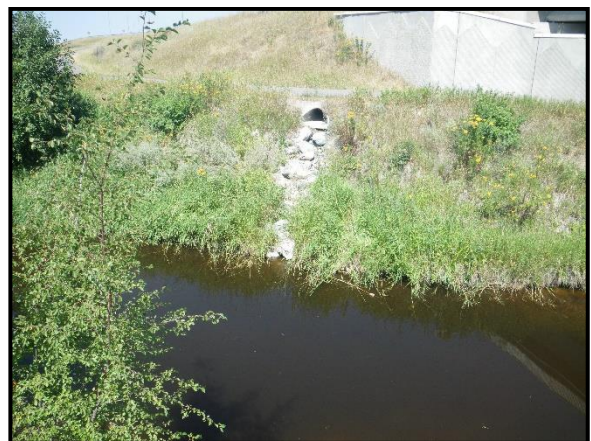
Additional Photo 6: Stabilized culvert outlet on the upstream end of the project area.
