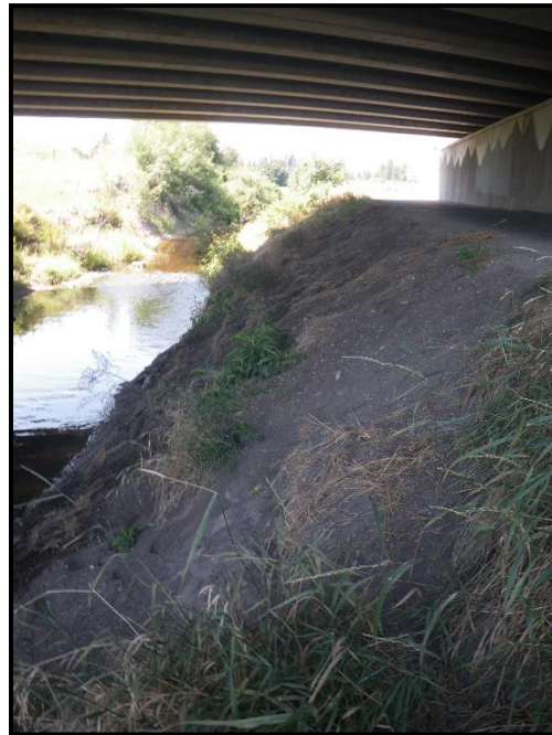
Additional Photo 9: Looking upstream at eroding bank EBL 2 showing bank sloughing and loss of vegetation.
