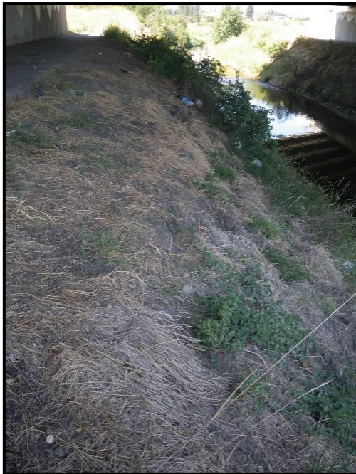
Additional Photo 8: Looking upstream at eroding bank EBR 2 showing bank sloughing and loss of woody vegetation.
