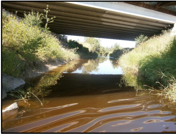
Survey Photo 27: T4: Looking West from creek.
