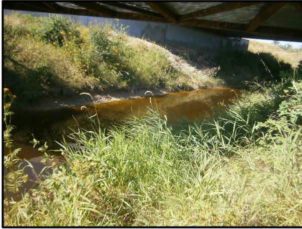
Survey Photo 25: T4 Left: Looking West upstream.
