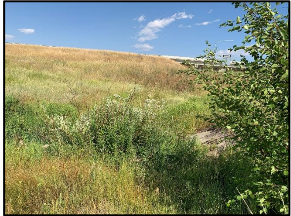
Survey Photo 8: T1 Right looking east downstream.
