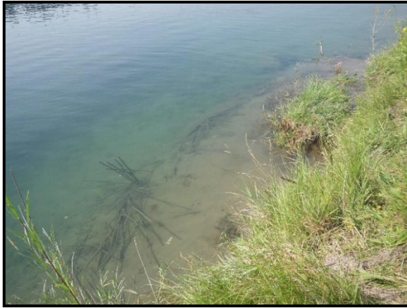
Additional Photo 1: Fascine underwater at T-1.
