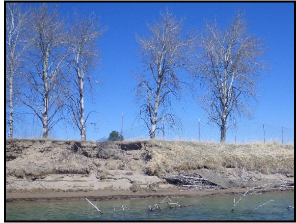
Additional Photo 2: Bank Erosion and fence entrapment at T-1.
