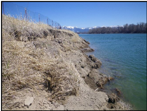
Additional Photo 3: Looking downstream (East) from T-2 at bank erosion. Note the absence of the fascine.
