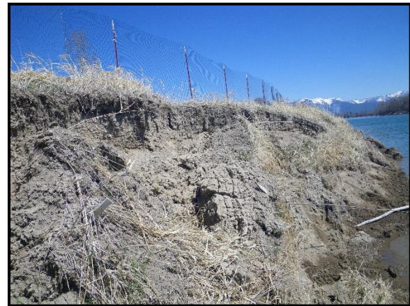
Additional Photo 2: Bank Erosion and fence entrapment at T-1.
