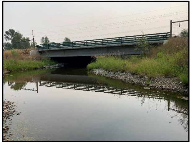
Survey Photo 22. T4 looking East downstream from middle creek.
