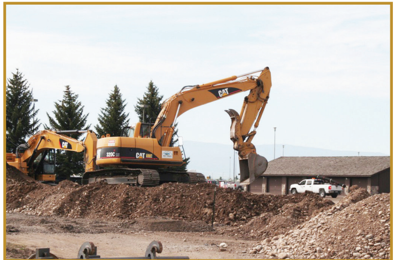
Figure 4: Construction at Bozeman Yellowstone International Airport
