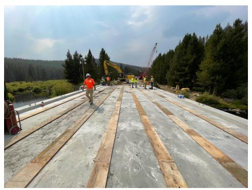
Figure 5: Keyways with top forming
