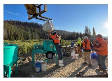
Figure 2: Sack of dry mix being added to the mixer
