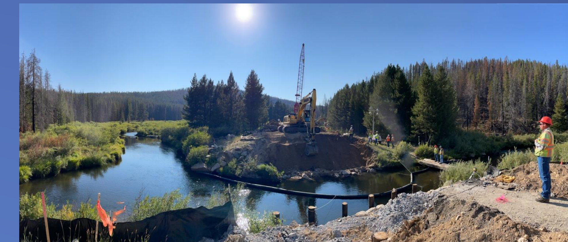
Demolition and Site Preparation
