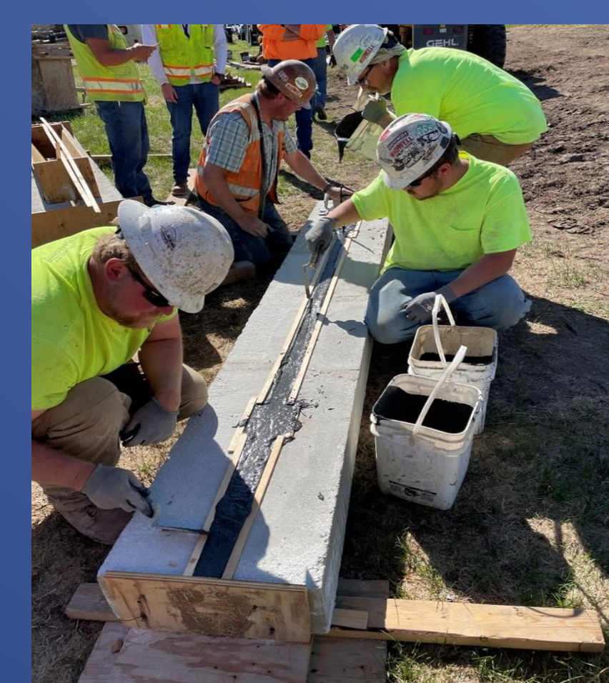
UHPC Placement in Pile Cap and Keyway
