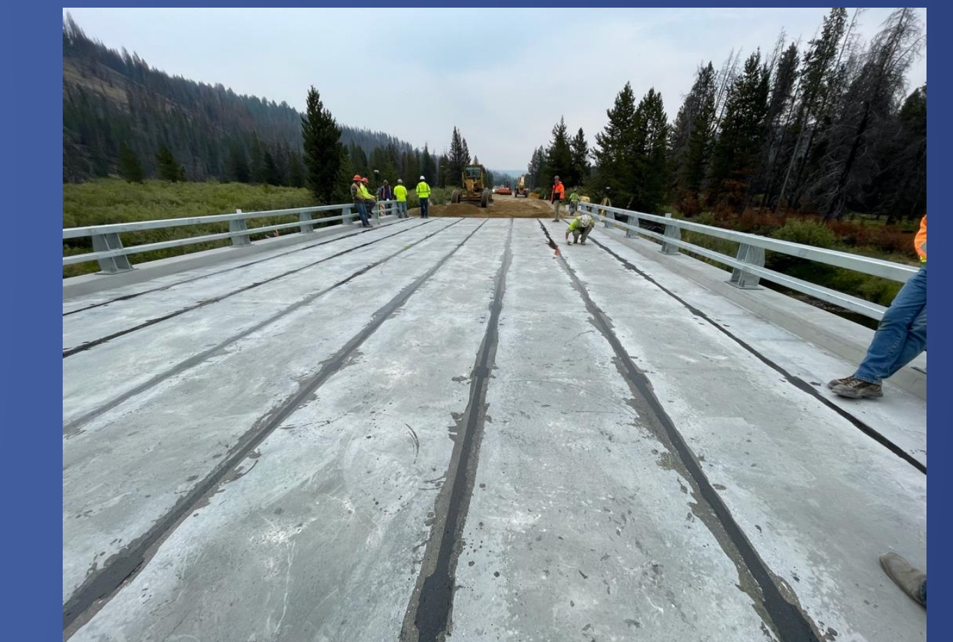
Finished Bridge with Epoxied Keyways
