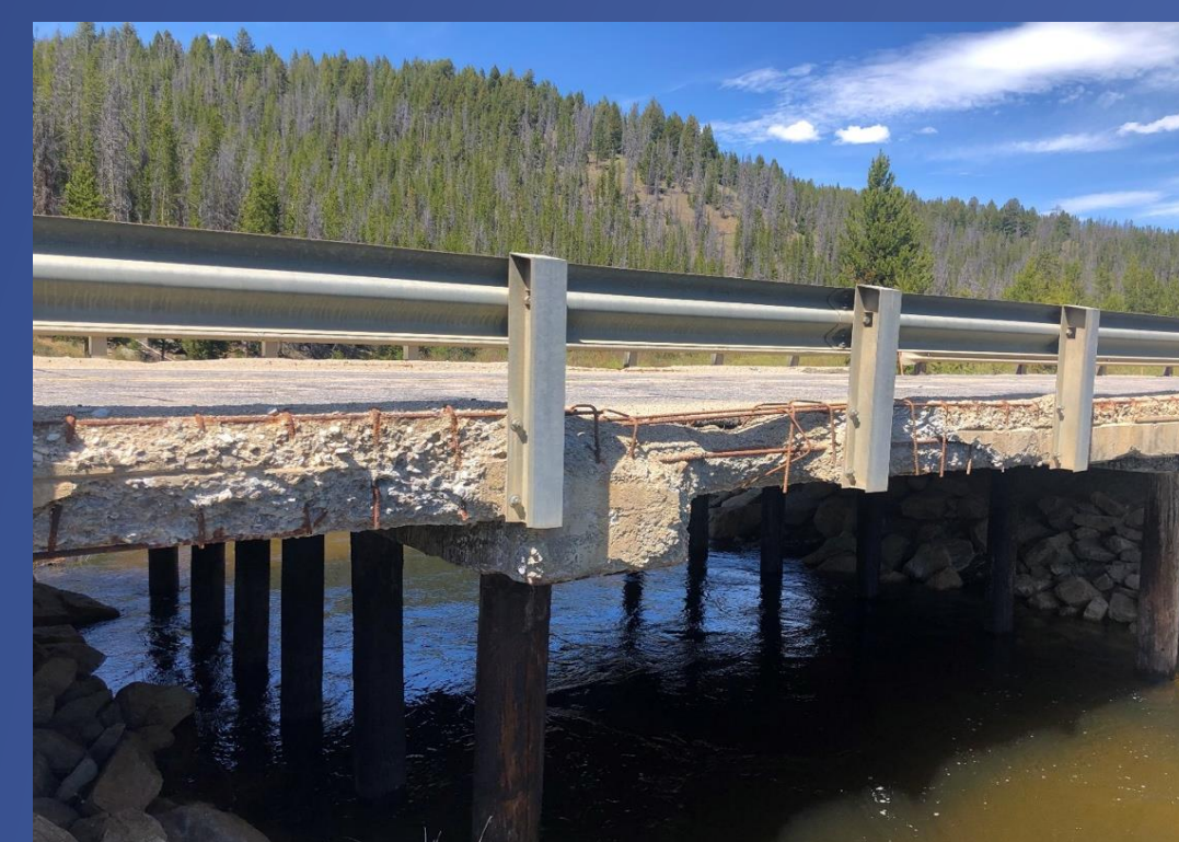
One of existing Trail Creek Bridges
