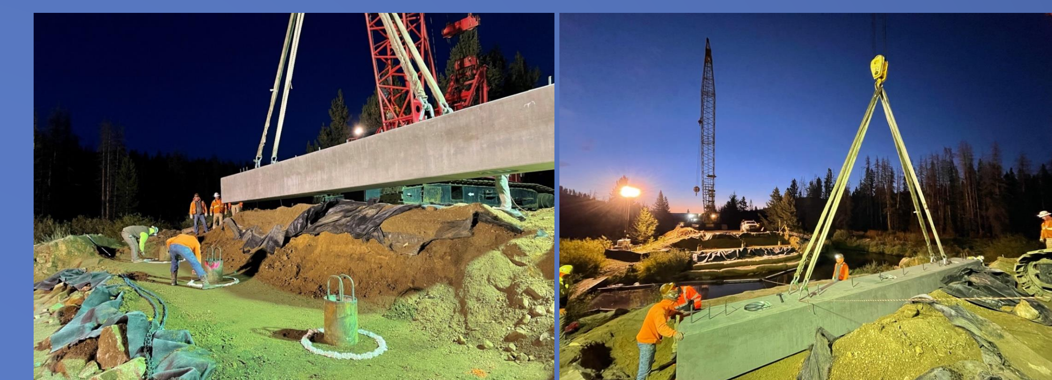
Pile Cap Placement
