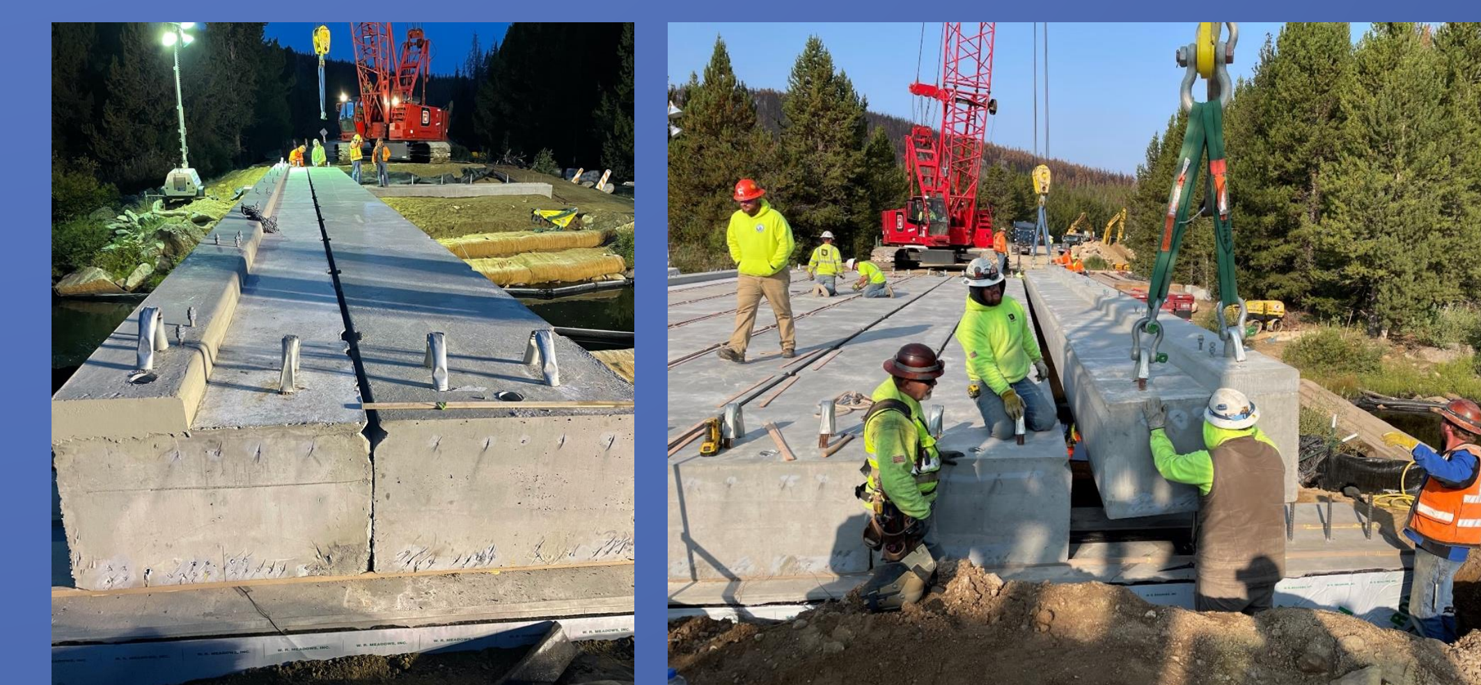
Placement of Beam/Deck Elements
