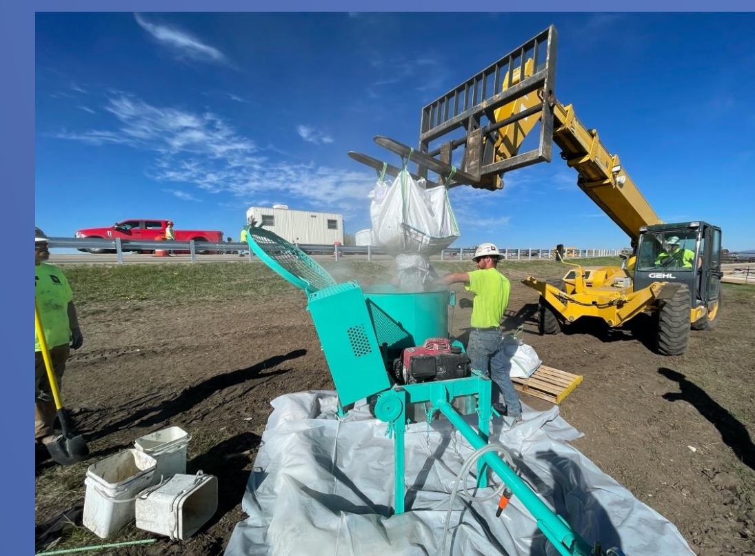
UHPC Batching/Mixing
