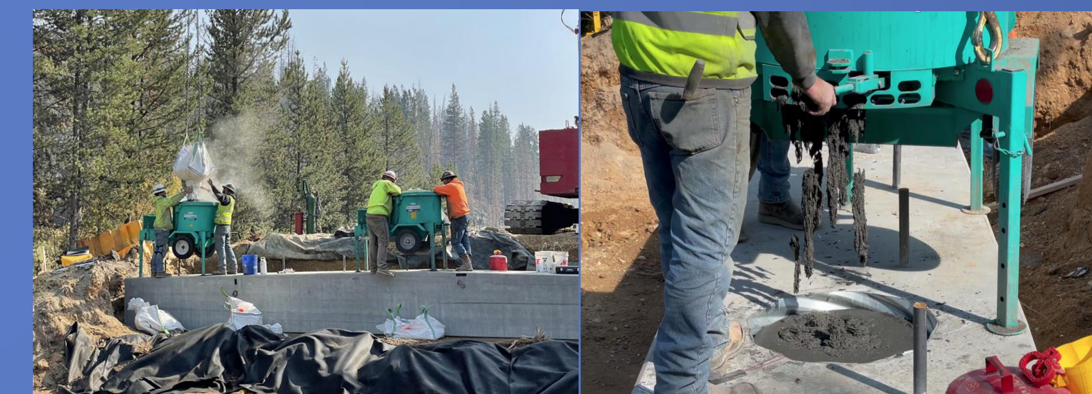
UHPC Placement in Pile Caps
