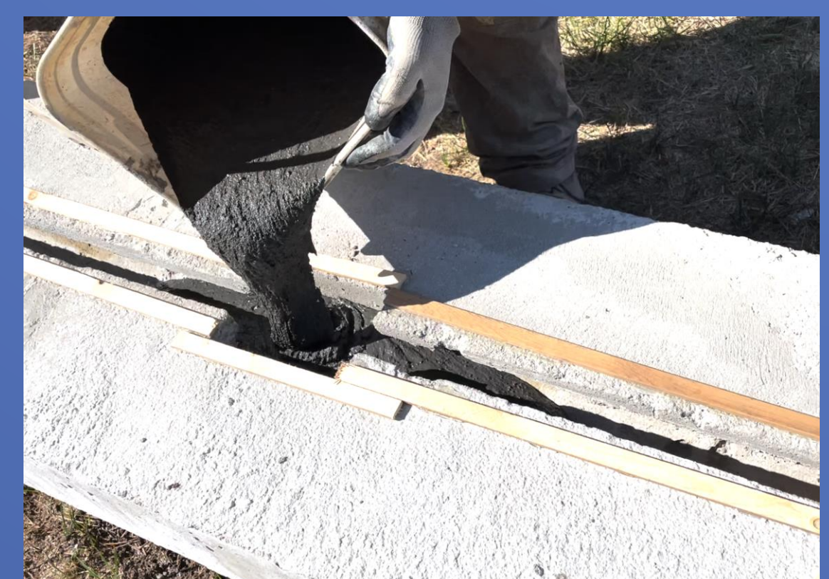
UHPC Placement in Pile Cap and Keyway
