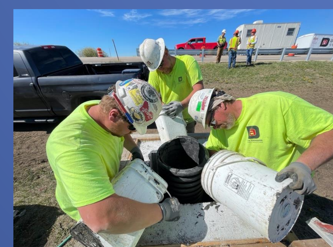
UHPC Placement in Pile Cap and Keyway
