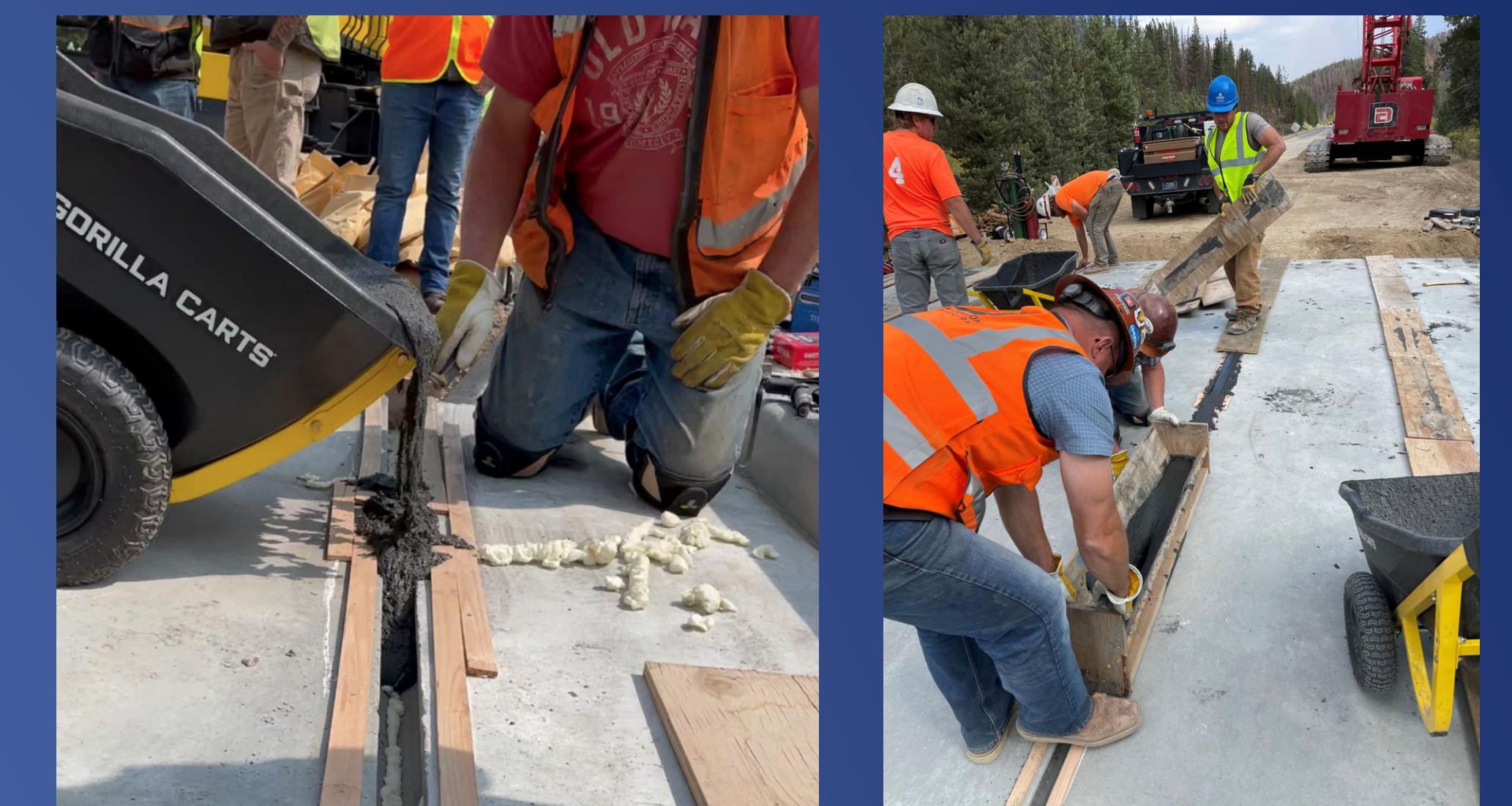
MT-UHPC Placement
