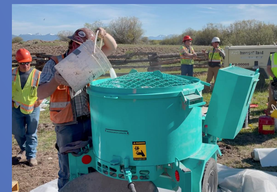
UHPC Batching/Mixing
