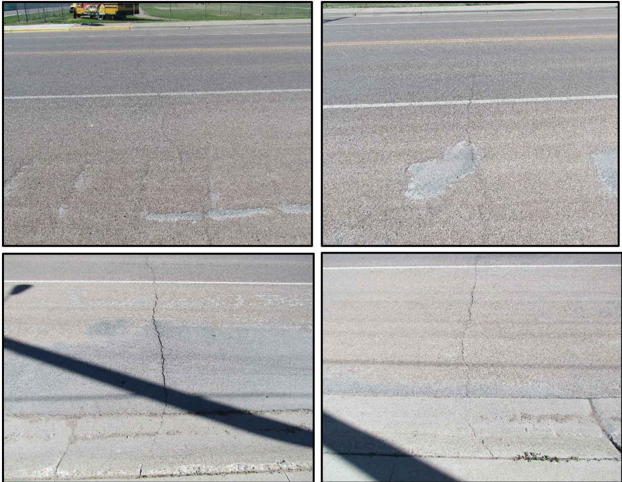
↑ This distress was noticed near the Riverview Boulevard intersection and are being highlighted because of how the crack continues from the plant mix into the concrete, suggesting an issue in the base.
