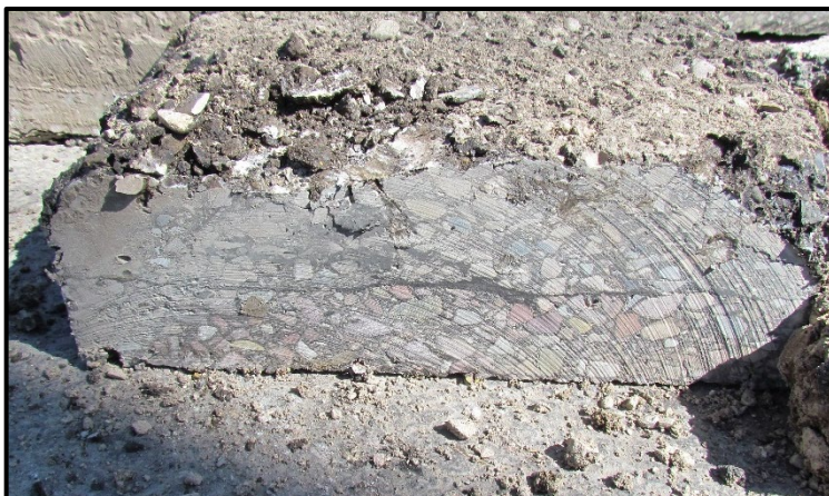
↑ This distress was noticed near the Riverview Boulevard intersection and are being highlighted because of how the crack continues from the plant mix into the concrete, suggesting an issue in the base.
