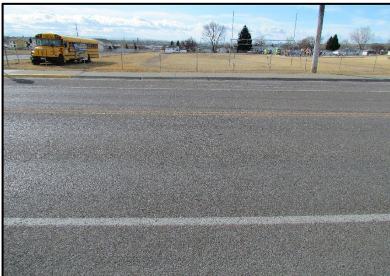
← Transverse view of pavement.
