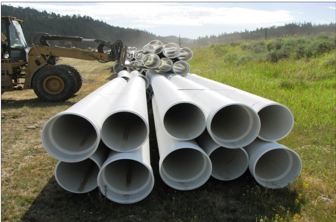
↑↓ Contech A-2000 pipe is delivered on-site.
