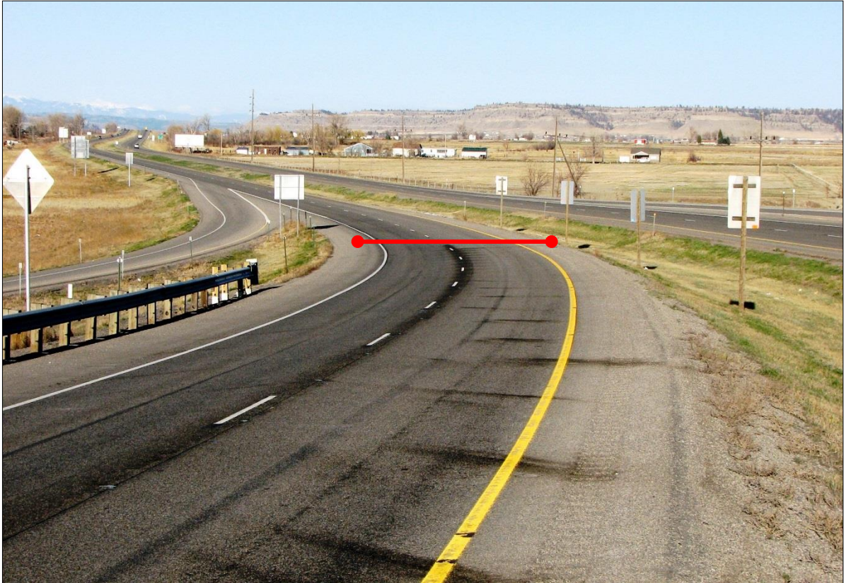
↑ View west of eastbound approach showing the delineation of the beginning of the spray nozzle section (red bracket).
