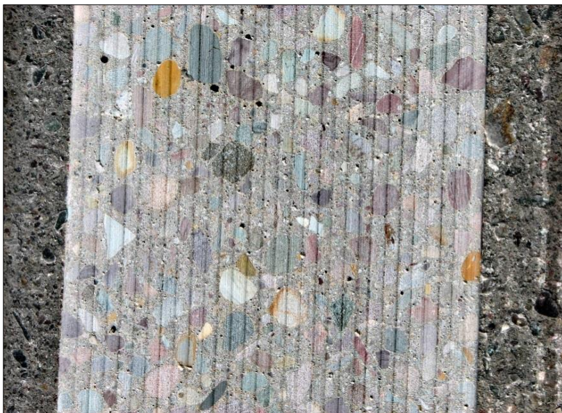
← Close-up of diamond grind. Groove relief represents a quality cut and clean definition.
