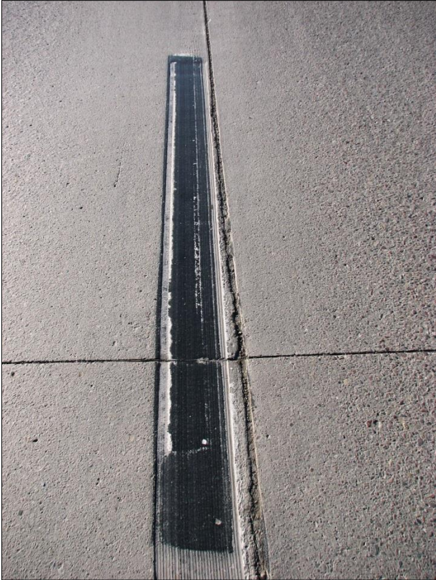
← Representative image of the contrast stripe with almost 100% of the top white stripe removed.
