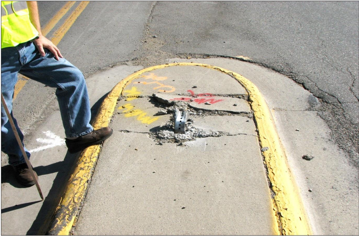
↑ ↓ Condition of the lane divider after two sign impacts. Location of the original sign placement (yellow arrow). Yellow circle will approximate location of new sign base.
