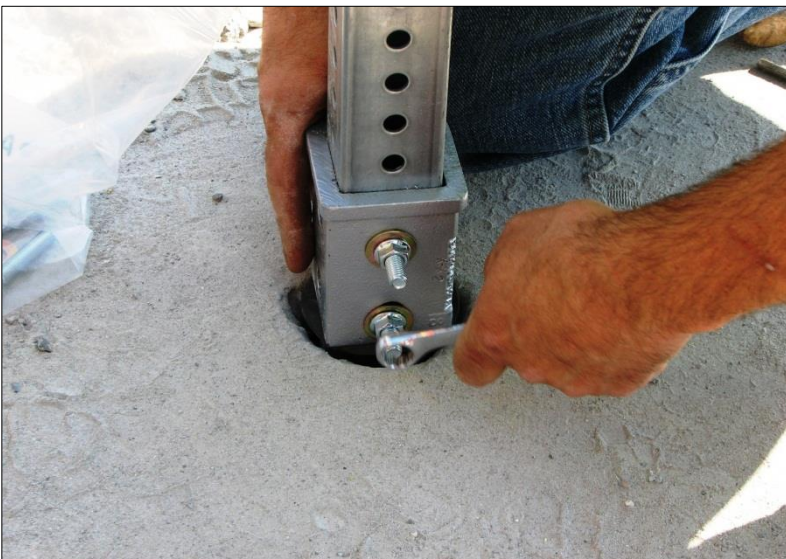
← Round head socket cap screws are set parallel through the sign base and Break-Out and tightened firmly.
