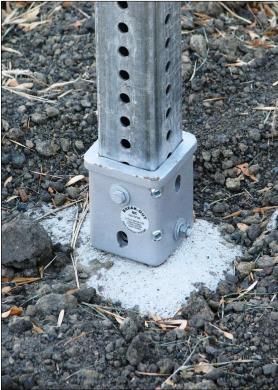
← Close-up of 2.5" diameter, square post unit in concrete base.
