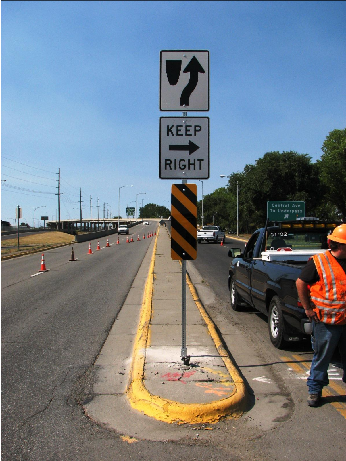
↑ Completed installation of the Break-Out Square Post coupler (view west).
