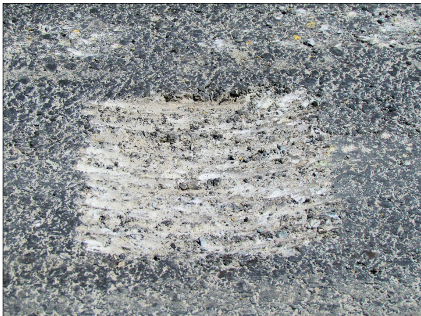
← Close-up of rectangular style rumble strip prior to seal and cover.
