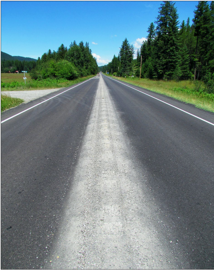
← View of completed pass of CLRS grind application.
