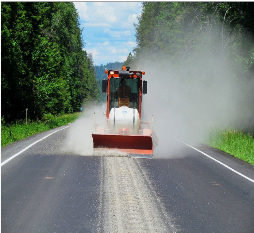
← Cleaning consisted of using a fixed-blade and connected sweep broom to remove millings off the road.
