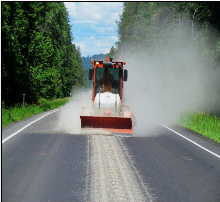
← Cleaning consisted of using a broom with a fixed blade to remove millings from the roadway.
