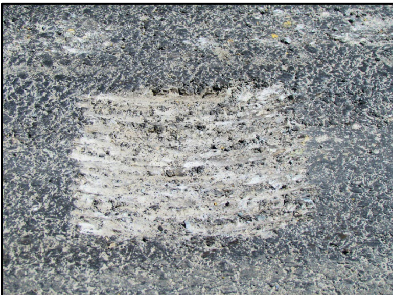
← Close-up of rectangular style rumble strip prior to chip seal.
