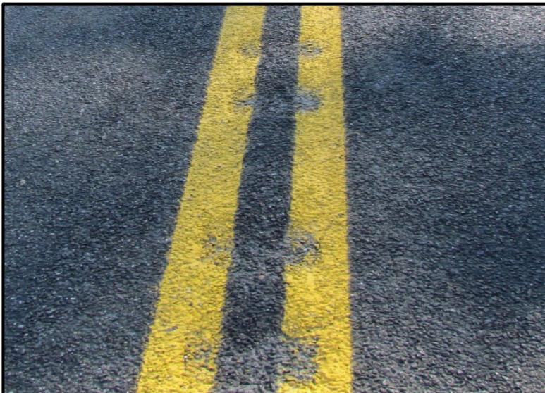
← Close-up of the CLRS after chip seal application.
