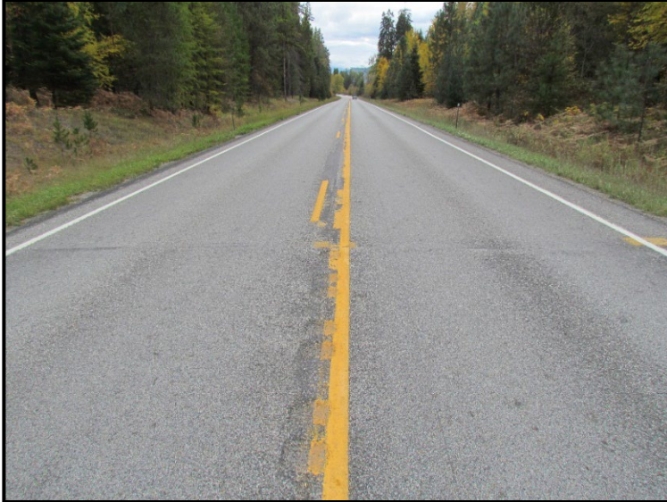
← RP 8.2, view east. Transition of TS1 and CS2.
