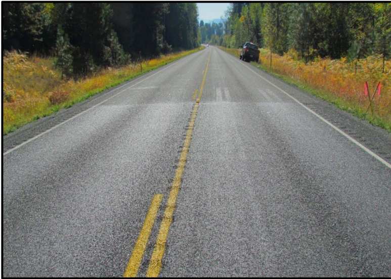
← Transition from TS1 to CS2 at approximate RP 8.2, view east.
