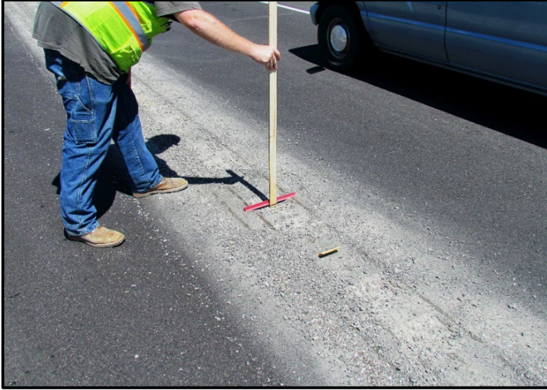
← The MDT inspector continuously monitored strip compliance during the project.
