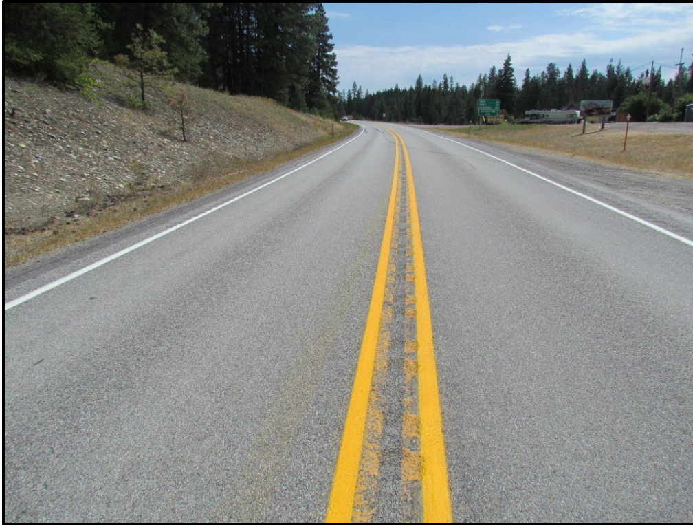
↑ RP 0.0, view east. Overview of TS1, centerline rumble strip section.
