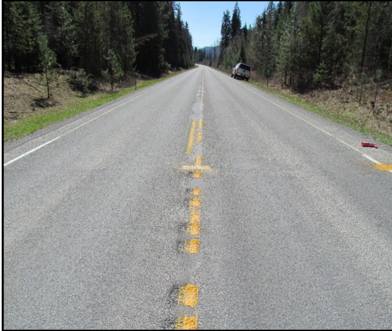
← Transition of sections TS1 & CS2, RP 8.2, view east.
