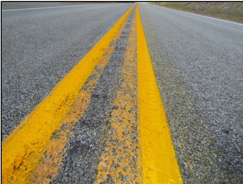
↑ RP 0.0, close-up view of TS1, centerline rumble strips.
