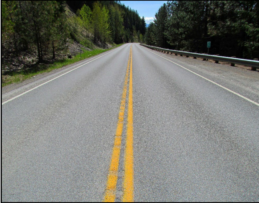
← Section TS1 at RP 5, view east.
