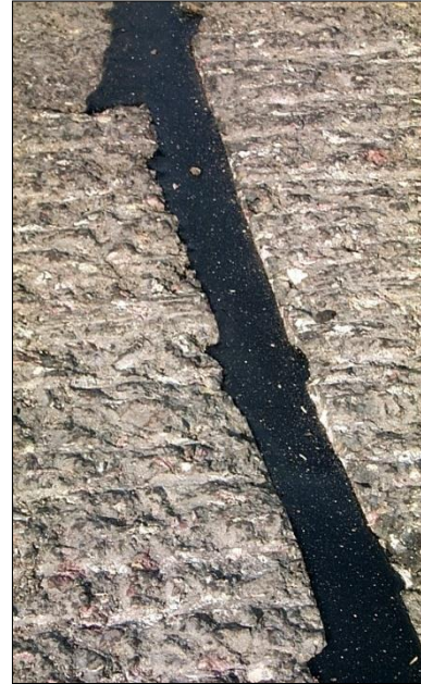
Sealed with Crafc Hot-applied Modified Asphalt Sealant
