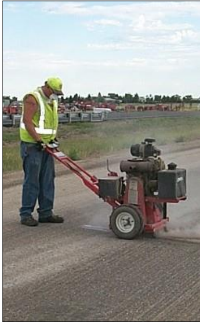
Grinding in process
