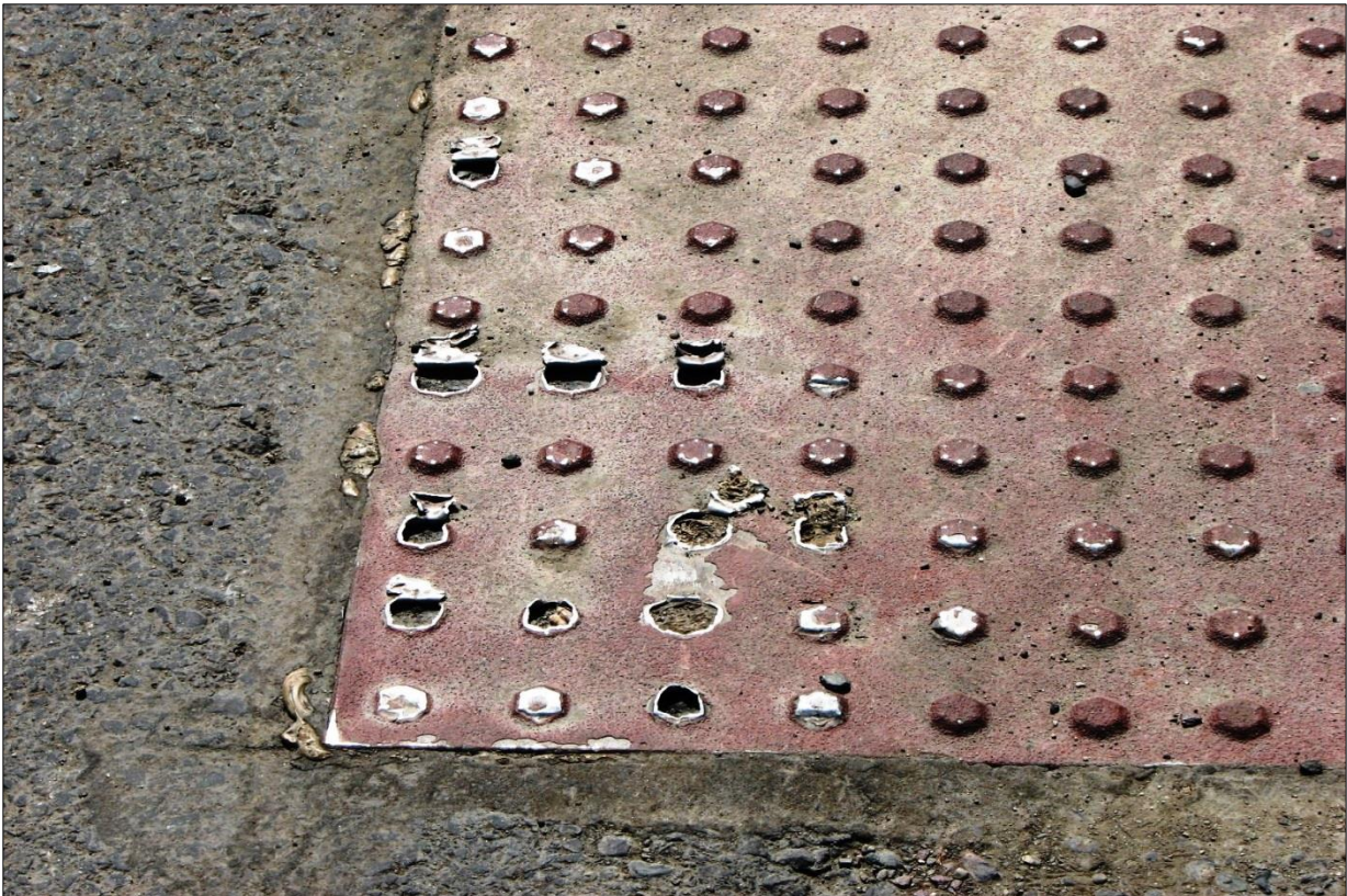
↑↓ Intersection of South Ave. and Clements Rd – West placement: Additional damaged panels by plow as defined in the area of the yellow circles. Lower image is a close-up of the damaged domes.
