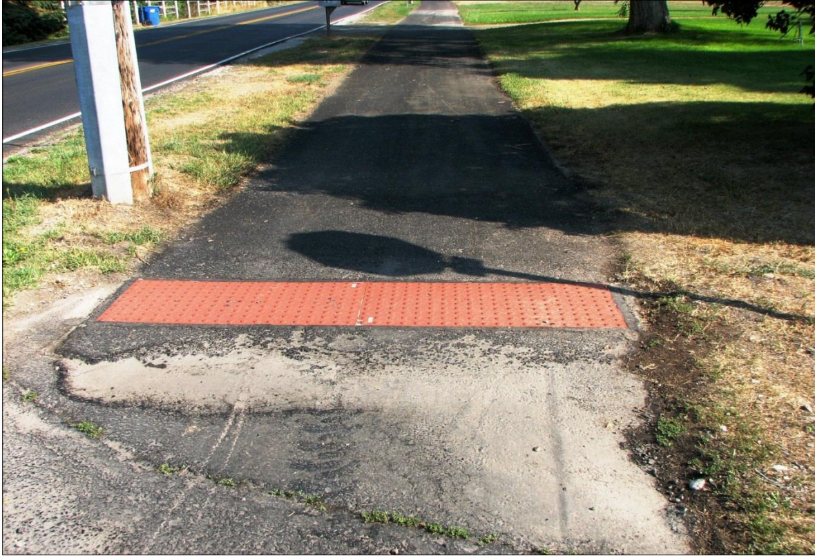
↑↓ Sample images of MetaDome DWD with paper removed after asphalt sealing.
