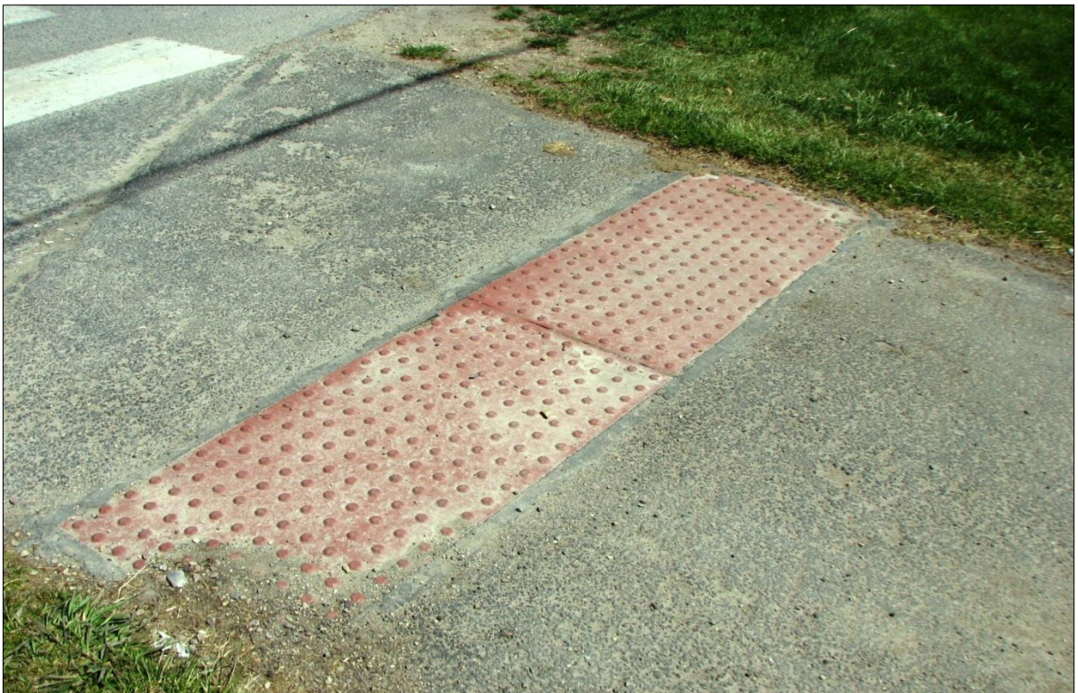
↑ ↓ Intersection of Mount Ave. and Clements Rd; east side of installation. The DWD's at this location were visually in good shape.
