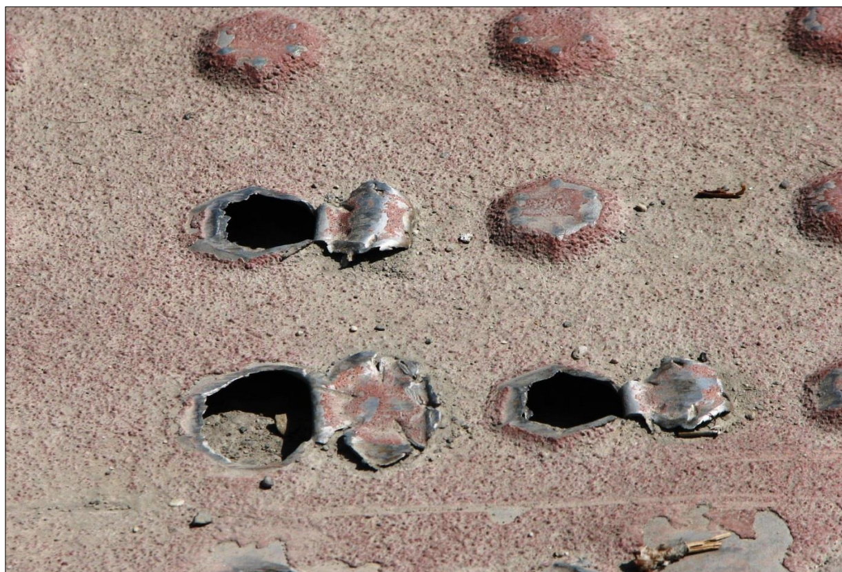
↑↓ Several close-ups of the damaged domes. Some domes were flattened; others completely removed or peeled back as seen in lower image. The peeled back domes may be a safety hazard since they are razor sharp to the touch.
