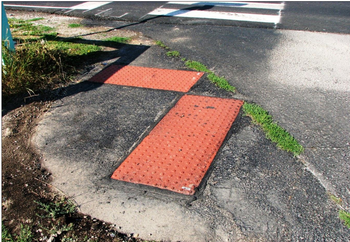
↑↓ Sample images of MetaDome DWD with paper removed after asphalt sealing.
