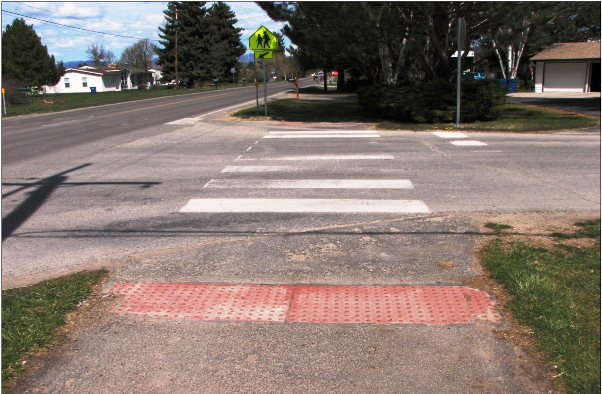
↑ ↓ Intersection of Mount Ave. and Clements Rd; east side of installation. The DWD's at this location were visually in good shape.
