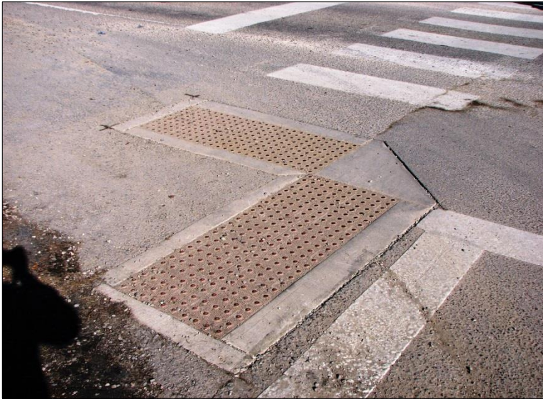
← Example of cast-iron DWD's replacing the damaged stainless-steel units.
