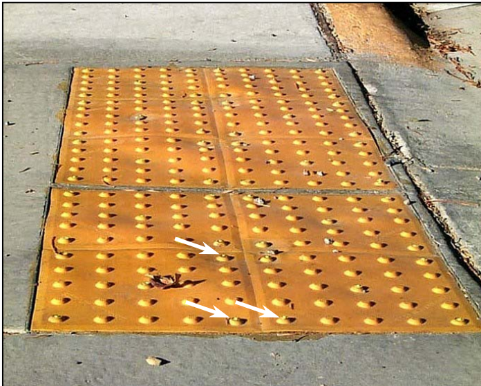
Installation 2: Side view looking east. Note the wavy texture of the mat.
