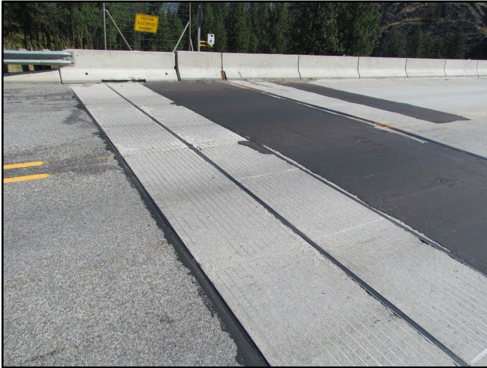
↑ West EWDM, transverse view. After the 2021 site visit, discussions were had about what to do with the damaged EWDM. Ultimately it was decided to replace the EWDM in a location approximately 50' west of the bridge end. To mitigate issues until replacement MDT Maintenance placed mastic over the damage to maintain safe crossing for vehicles.
