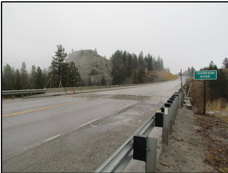
← View of fencing set up at the west EWDM. The main difference here is the use of the bridge as another form of deterrent. Because of this there only needed to be fencing panels on the wing walls.
