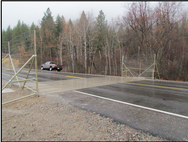
← View of the east EWDM that highlights how the wildlife fencing is used to fully restrict animal access to the wildlife free zone.
