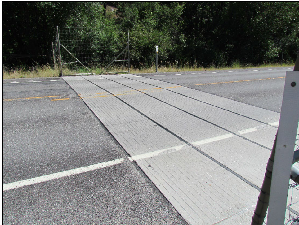
↑ East EWDM, transverse view. The EWDM in this location remains in good condition and operational.
