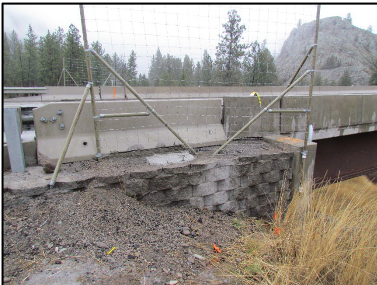
← View of the fencing anchored to the wing wall which in tandem with the west EWDM restricts animals from accessing the wildlife free zone by using the wing walls to bypass the EWDM.
