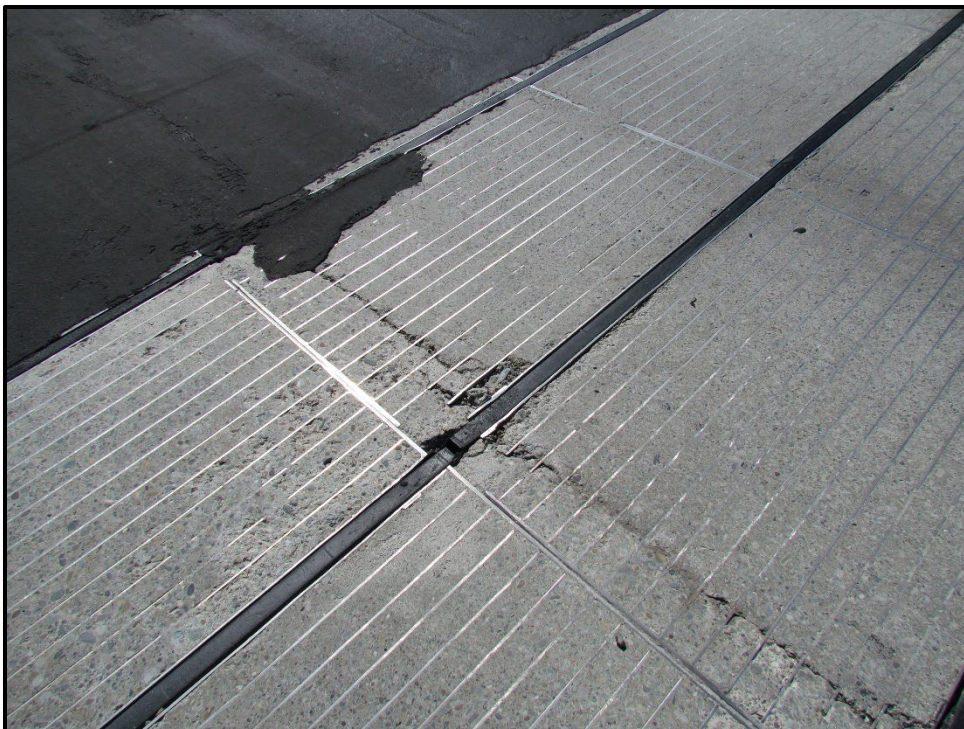
↑ West EWDM, close-up view. Damage at the concrete seam continues to worsen.
