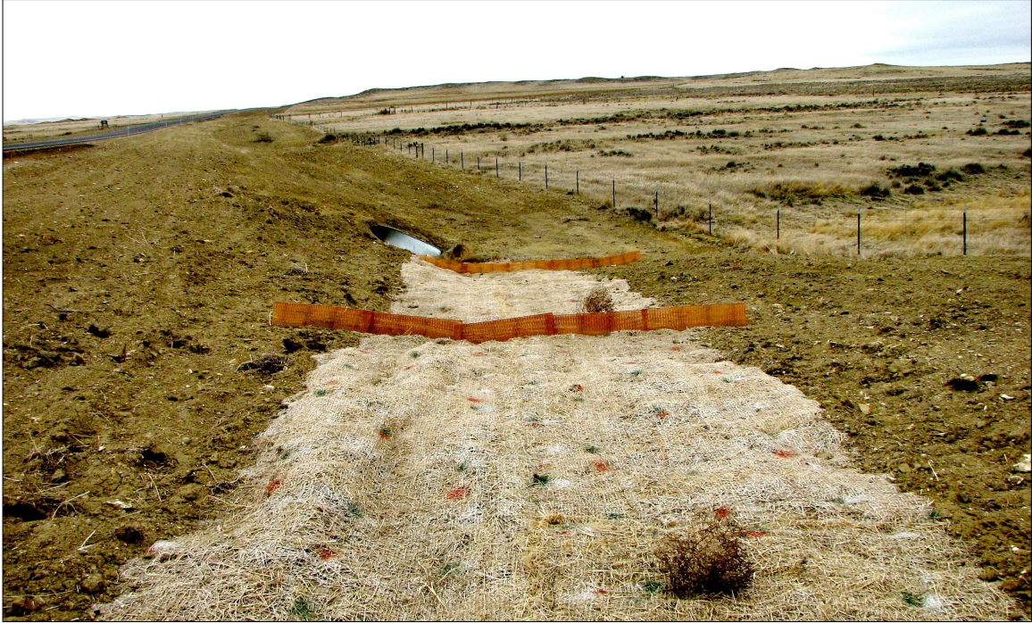
May 2008: Example of GeoRidge and erosion blanket lay-out on the Angela N & S project located in the Glendive District, highway 59 (P-18) approximate mile point 24; north of Miles City.
