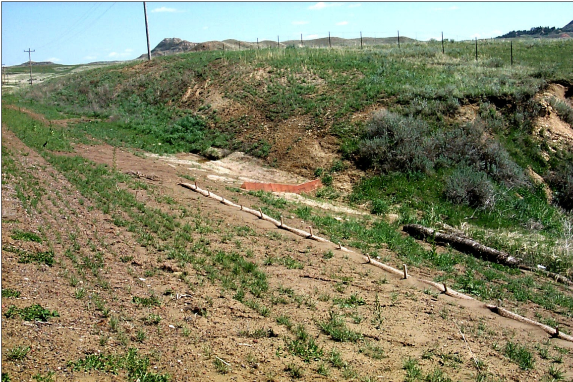
June 2007: This image shows the biodegradable PPB used conjunction with conventional wattles and erosion blankets.
