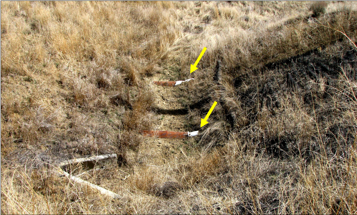
May 2008: Same site depicted in the previous image. Sand bags were placed to supplement the gaps in the berm sections (yellow arrows). It also appears that some of the accumulated sediment may have been removed and the PPB's cleaned and reset. Revegetation below the PPB's was well established.
