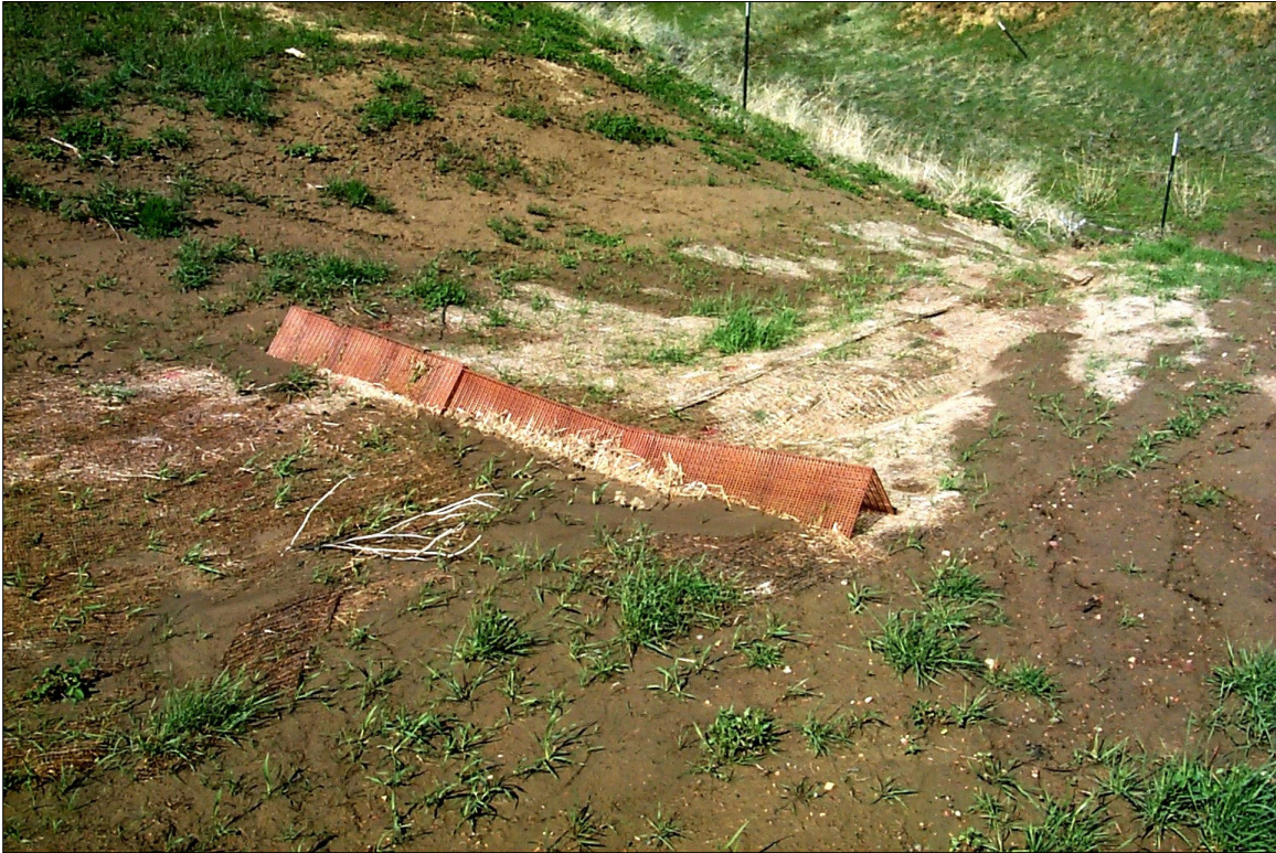
June 2007: Image representing the biodegradable PPB use in conjunction with an erosion mat.
