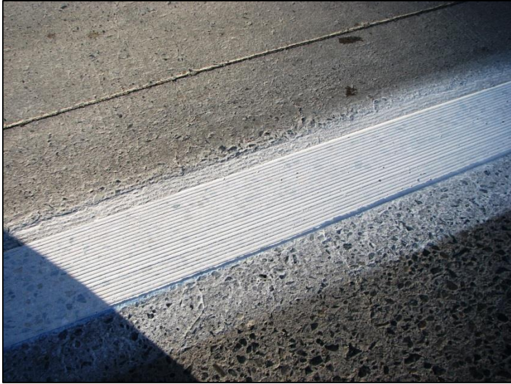
← Representative image of the grooved surface approximately 7" (17.78cm) in width.
