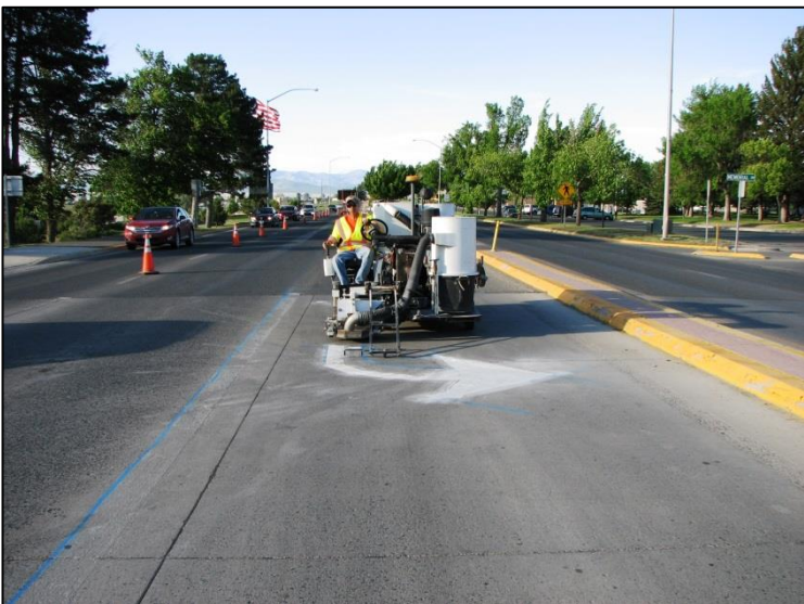
← Here the grooving machine starts the grinding of the arrow.
