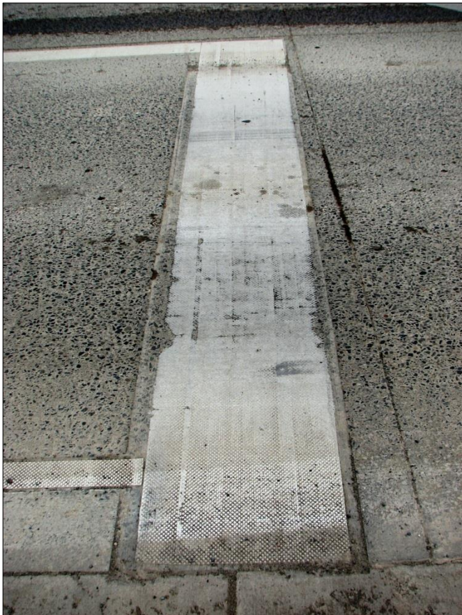
← ↑ General representation of continued pavement tape deterioration.
