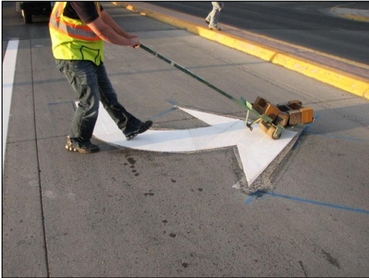
← An example of the weighted roller cart tamping an arrow.
