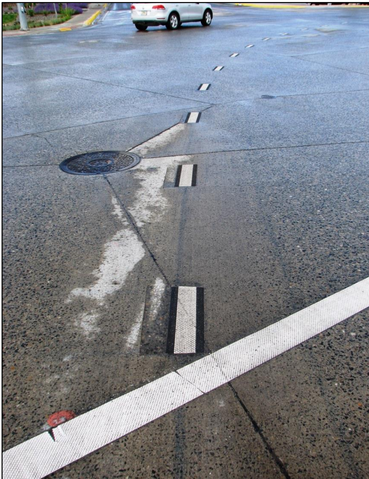
← Bordered contrast broken line markers were included on the site as lane dividers.
