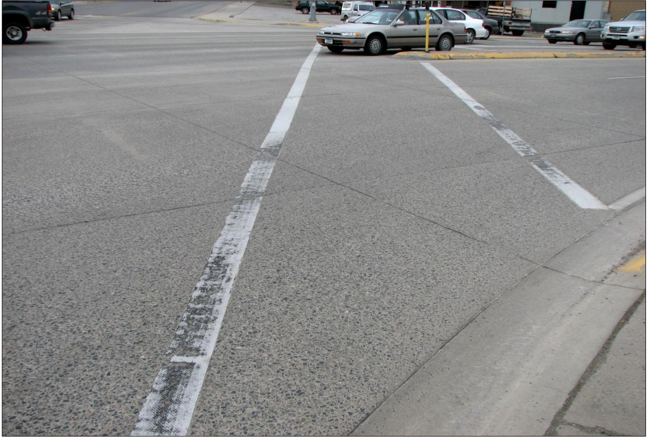
← ↑ General representation of continued pavement tape deterioration.
