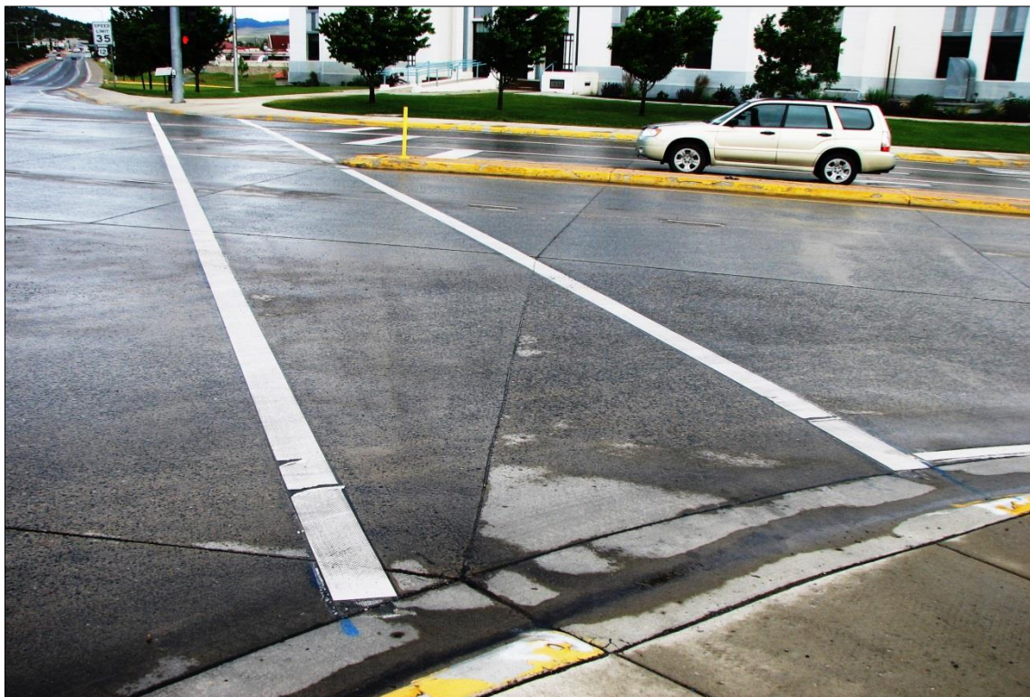
↓ Right turn from West Lyndale onto Last Chance Gulch: Turning movements are stretching and tearing the pedestrian lines.
