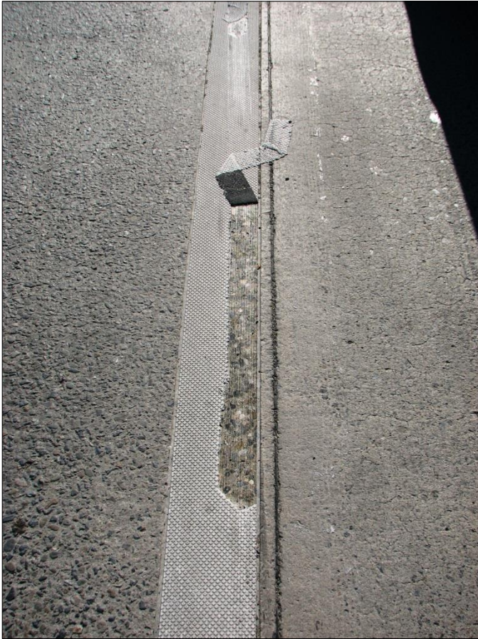
← Sample image of a friction tear most likely caused by sudden braking of a vehicle.
