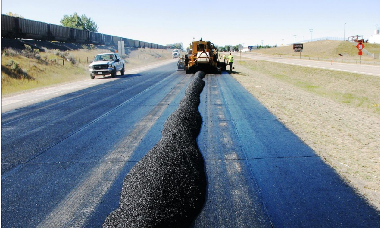
↑ Additional view of the paving process.
