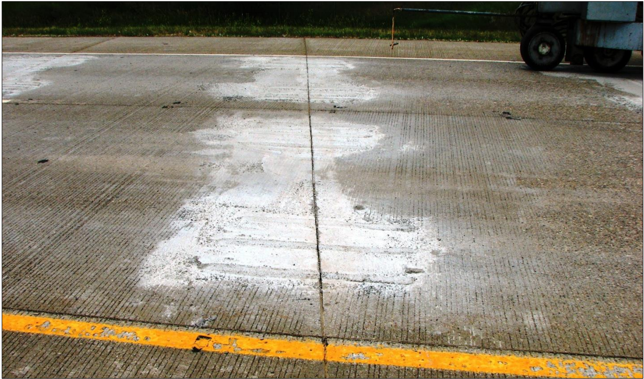
↑ Completed and patched dowel retrofit with applied curing compound.
