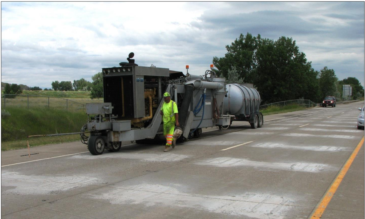
↓ Micro-grinding in process, first pass of the travel lane.
