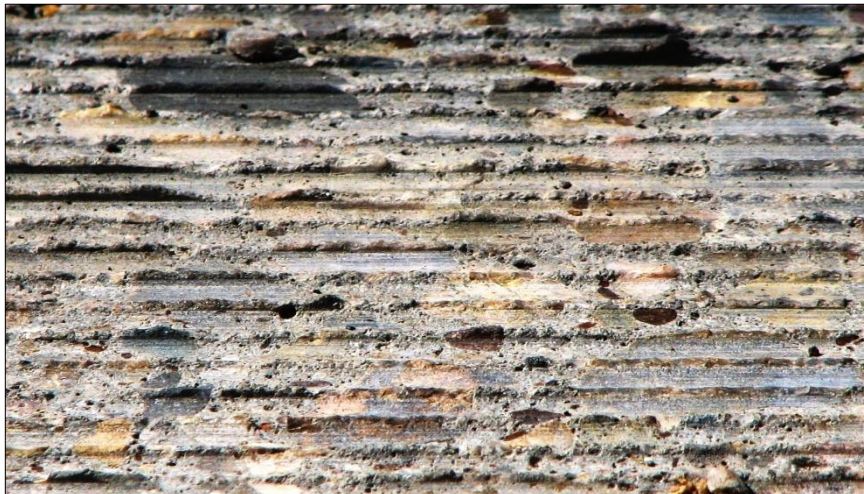
← Lateral close-up of the diamond grind. Blade width is approximately .25" (6.3 mm).
