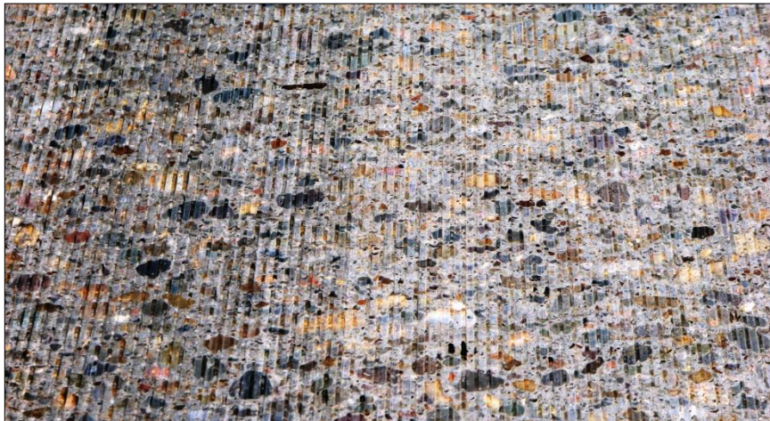
← Example image of the PCCP after grinding process.
