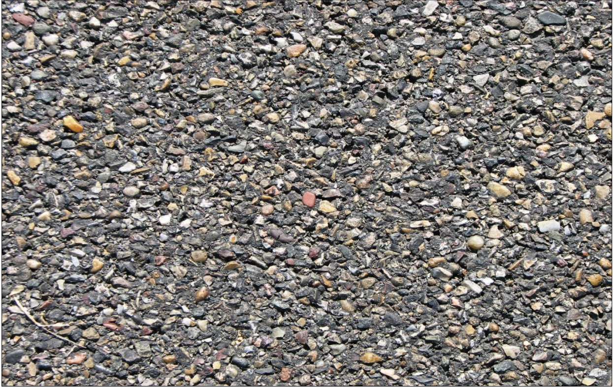
↑ ↓ Representative Images of PMS surface texture. No abnormal surface deformation noticed. No apparent bleeding or raveling is perceptible throughout the project. Polishing of aggregate minimum.
