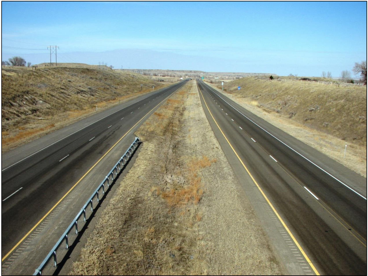
↑ Reference point 211: Overview of project looking east. As of April 2014 visual documentation portrays the combined PMS application and PCCP dowel retro-fit treatments as performing well.
