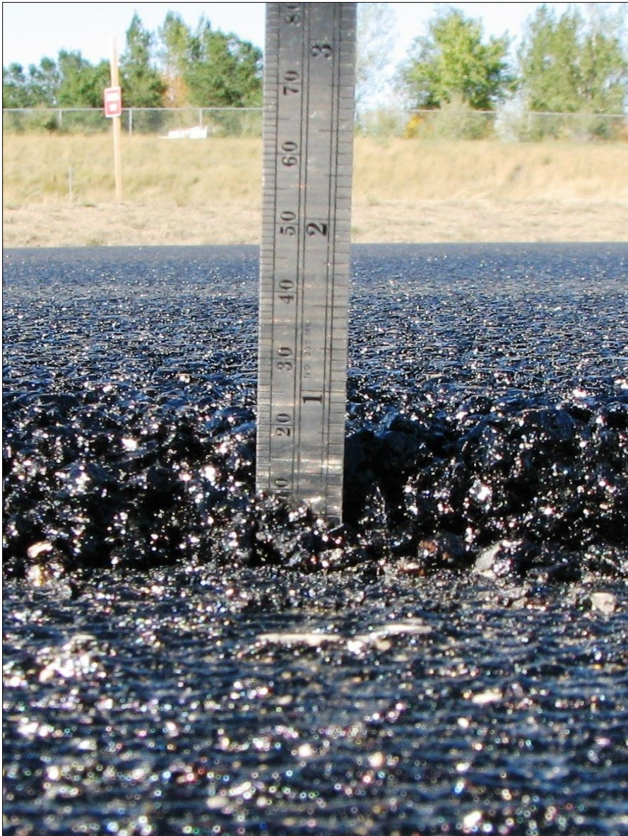
← Thickness of the PMS was specified at 16 mm (.625").
