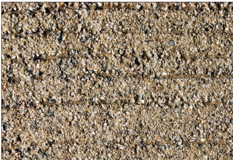
← Closer view of PPC texture in the wheel path.
