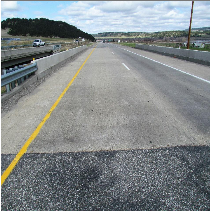
← Westbound passing lane; view west.
