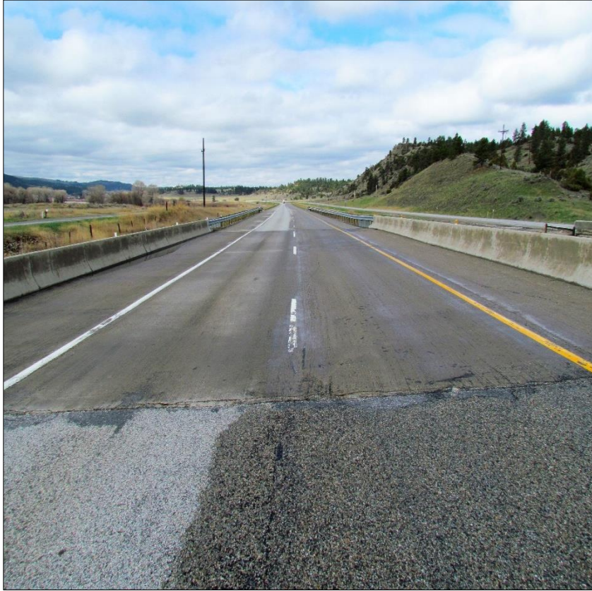
← Berry Creek eastbound; view west.
