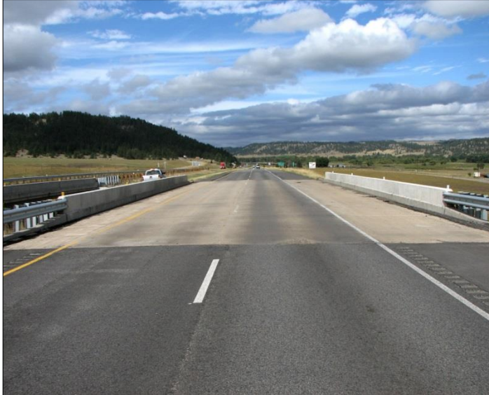
← Sep County Rd.: Westbound deck I-90; view west.
