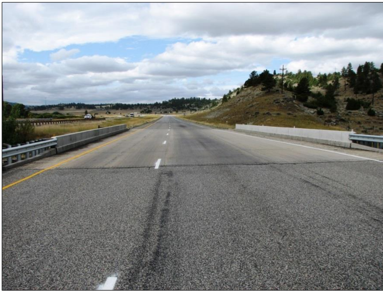
← Berry Creek Structure Westbound I-90: View west.
