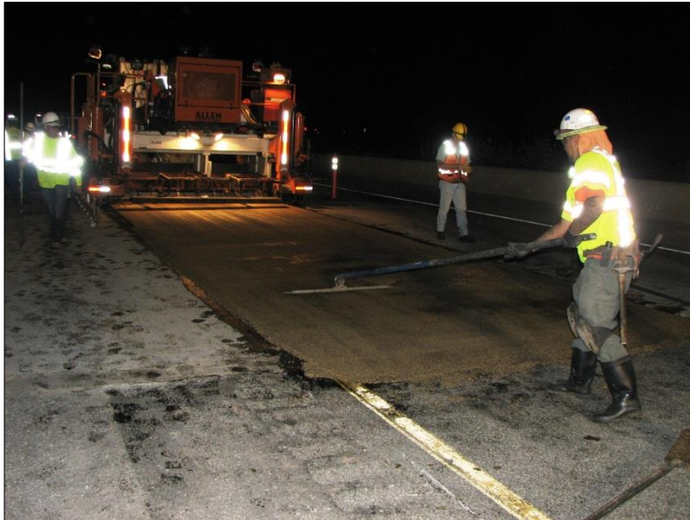
← Another image showing the workman applying a float to the PPC.
