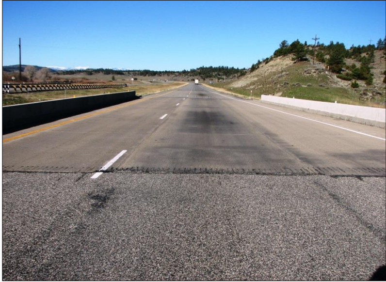
← Berry Creek Structure Westbound I-90: View west.
