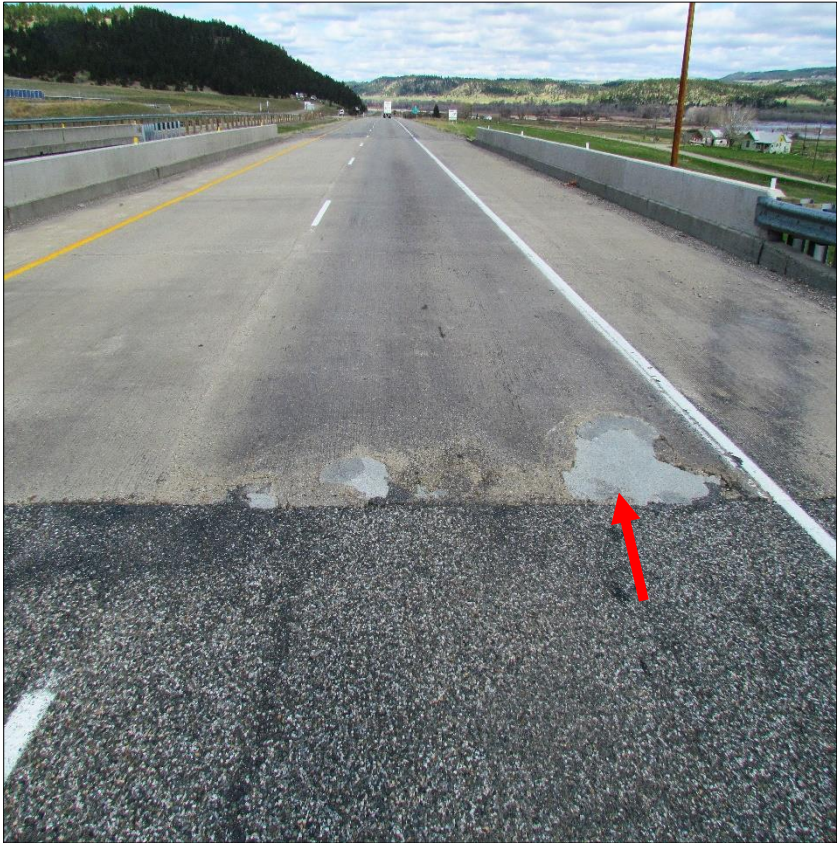
← Westbound travel lane; view west.
