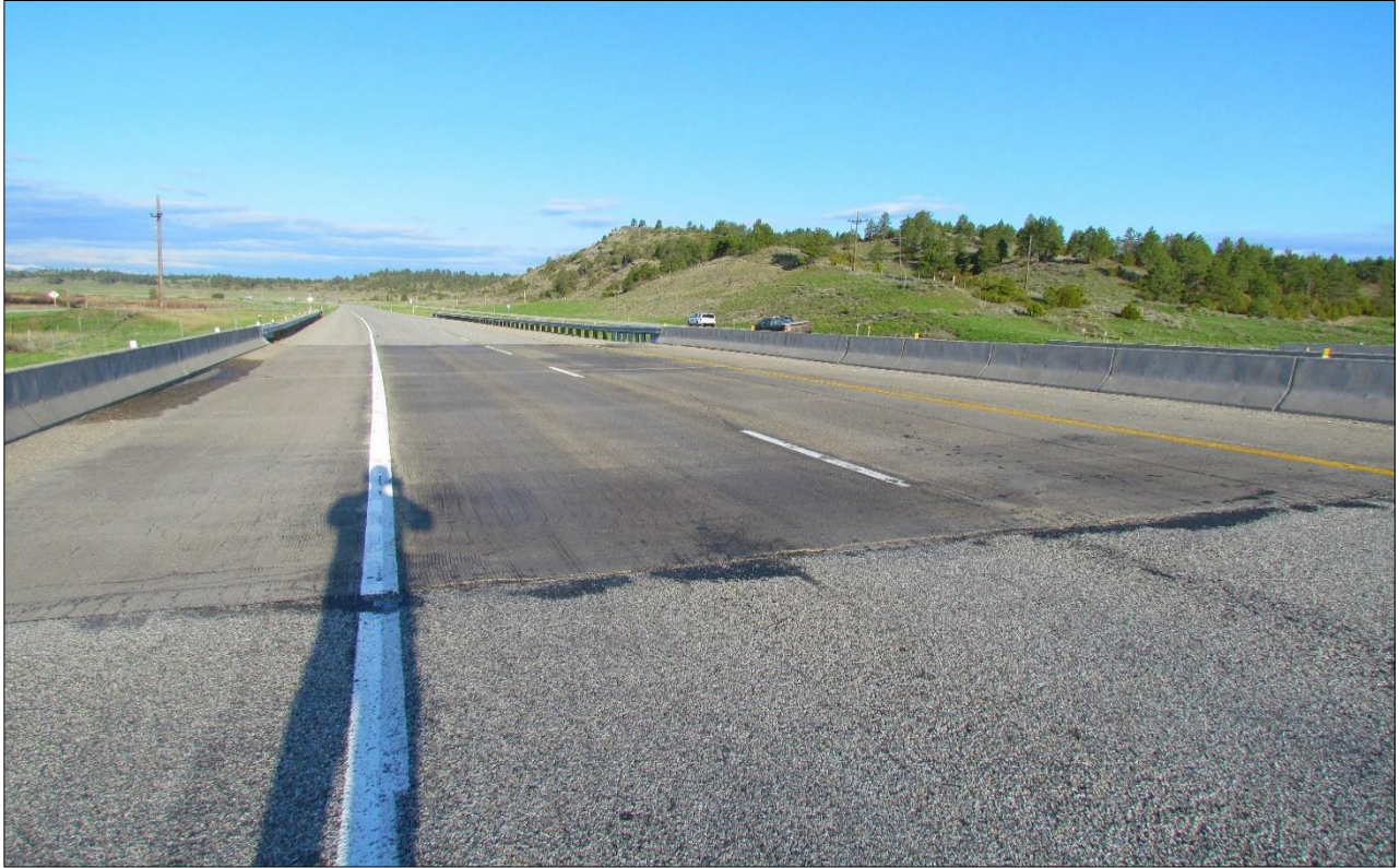
↑ East end of Berry Creek Rd. eastbound structure (view west).
