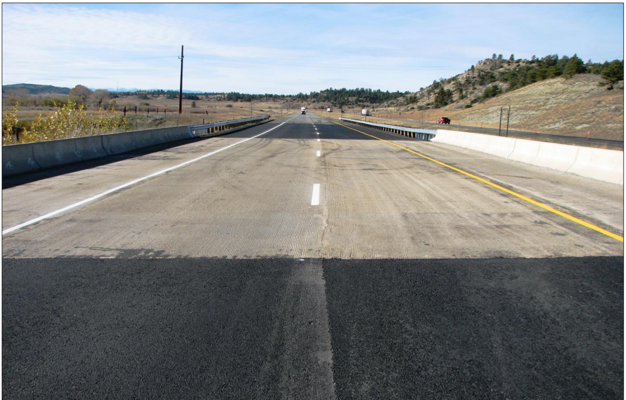
↓ Berry Creek Structure – Eastbound I-90: View west.
