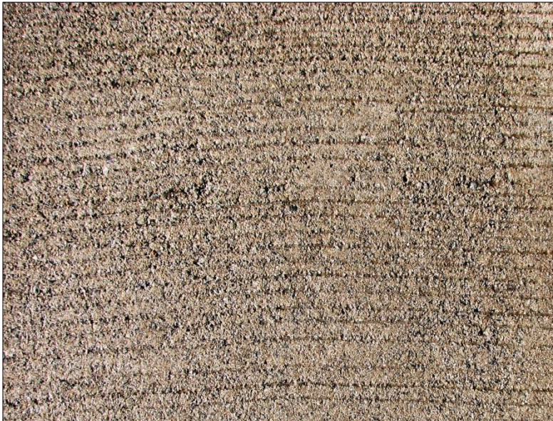
← Surface textures in both lanes appeared to be in good condition since installation.
