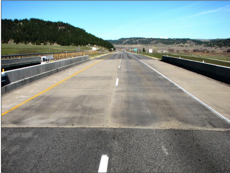
← Sep County Rd.: Westbound deck I-90; view west.
