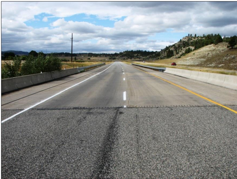
← Berry Creek Structure Eastbound I-90: View west.
