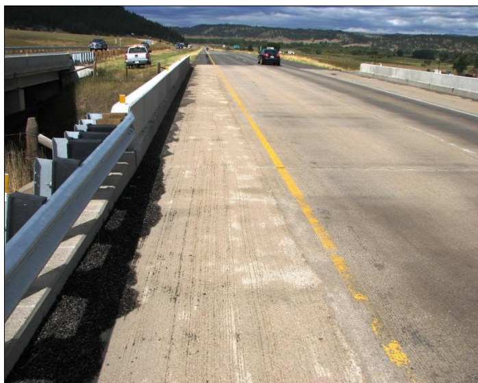
← Additional plow abrasion is apparent on the deck shoulder; predominately on the south side.
