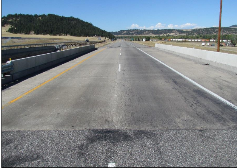
← SEP County Rd: Westbound; View West.
