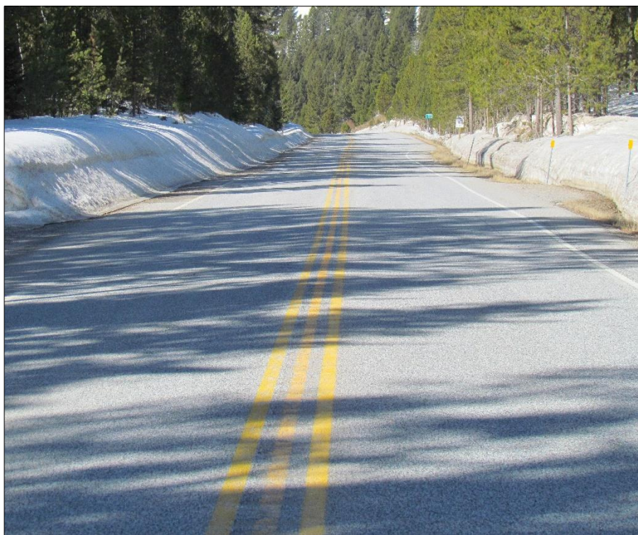
← Representative image of project during 2020 inspection. East end, view west.
