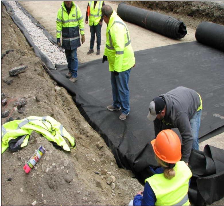
← The geosynthetic lining the trench is placed over the SSDL.
