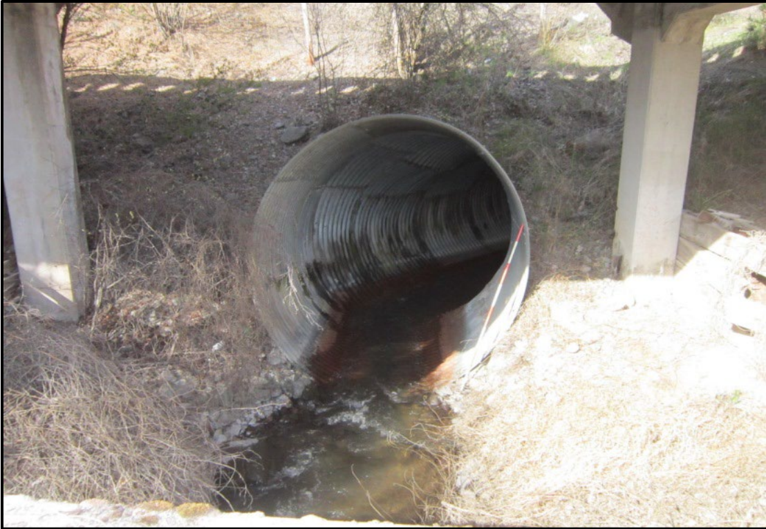
↑ Upstream culvert inlet view, east end.
