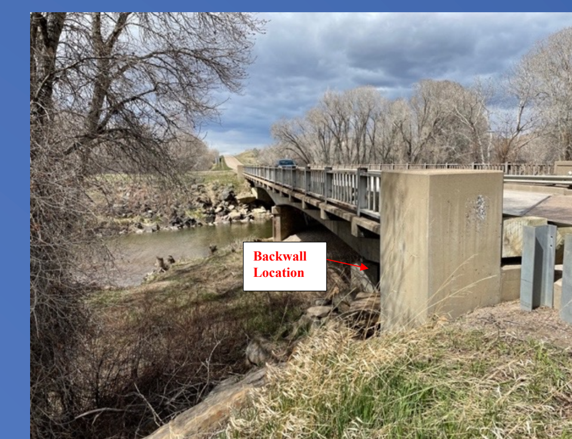
Backwall Location on Bridge
