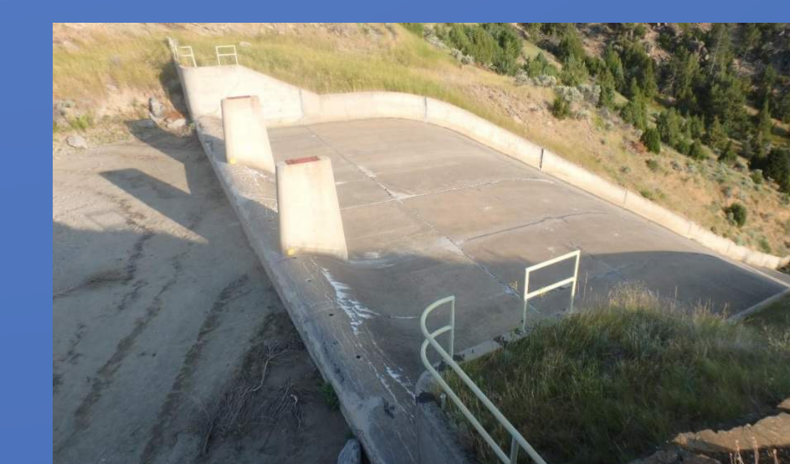
Ogee of Dam
