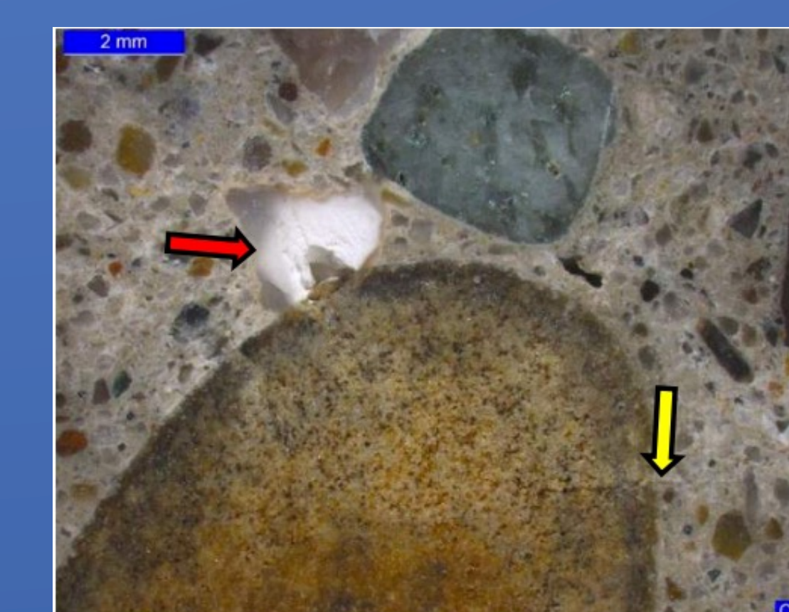
Core from Chute Showing ASR Gel Deposits
