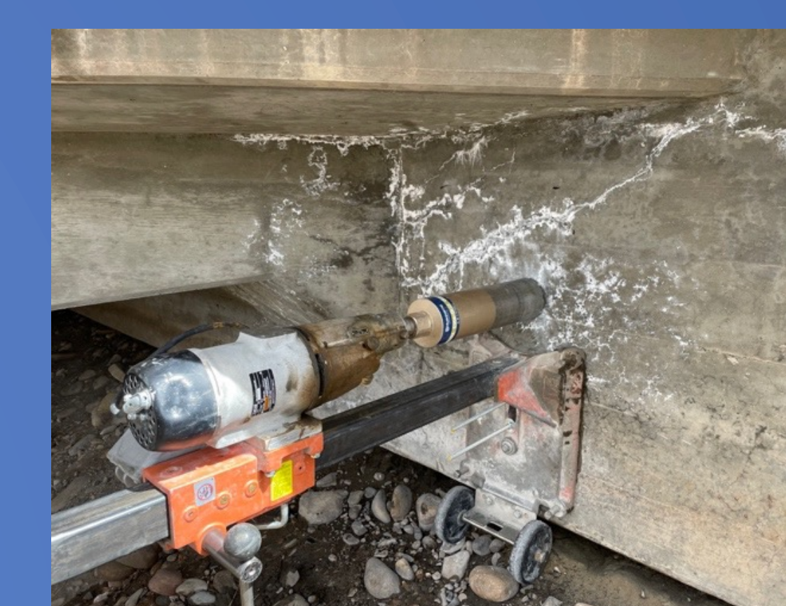
Backwall Being Cored
