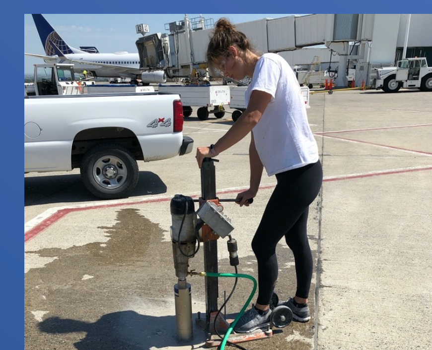
Coring of Site 1
