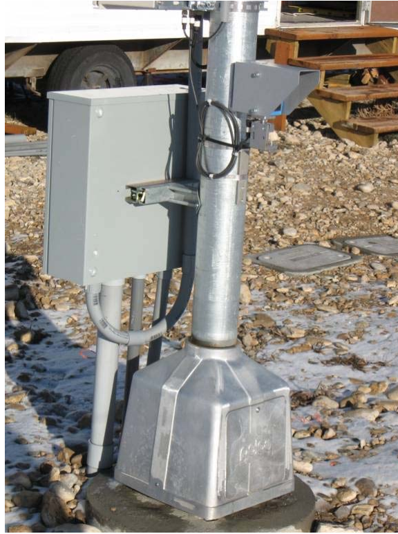
Figure 3.10: System 5 (Calonder Energy 1) (Photo: Marcel Huijser, WTI/MSU).
