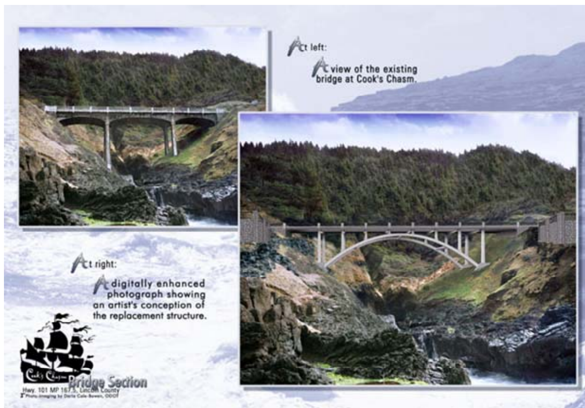
Figure 3: The Cooks Chasm Bridge. Source: Lea Ann Hart-Chambers, ODOT.
